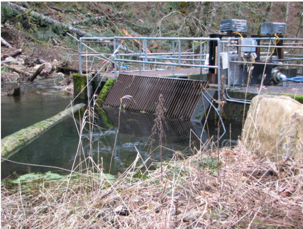
Photograph 2. Upstream View of the Intake
