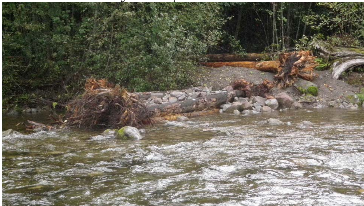
A series of structures were placed to reduce flow on river left ST#5
