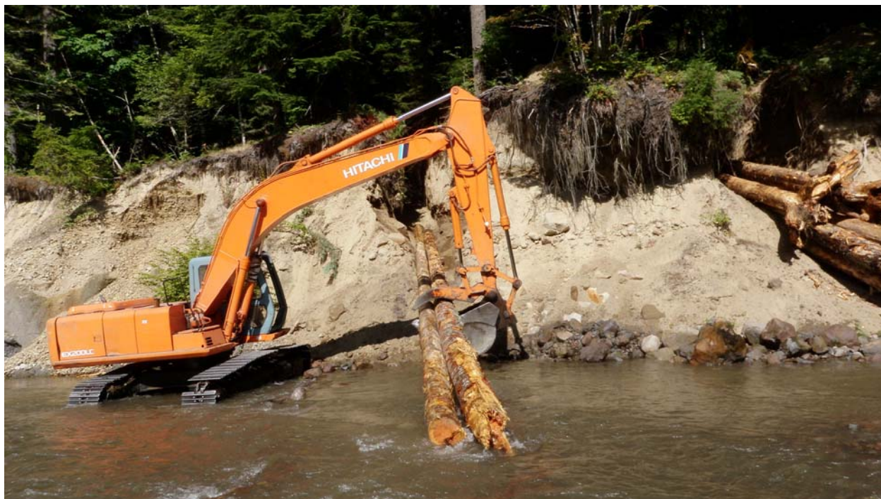
Excavator placing logs into banks ST#10
