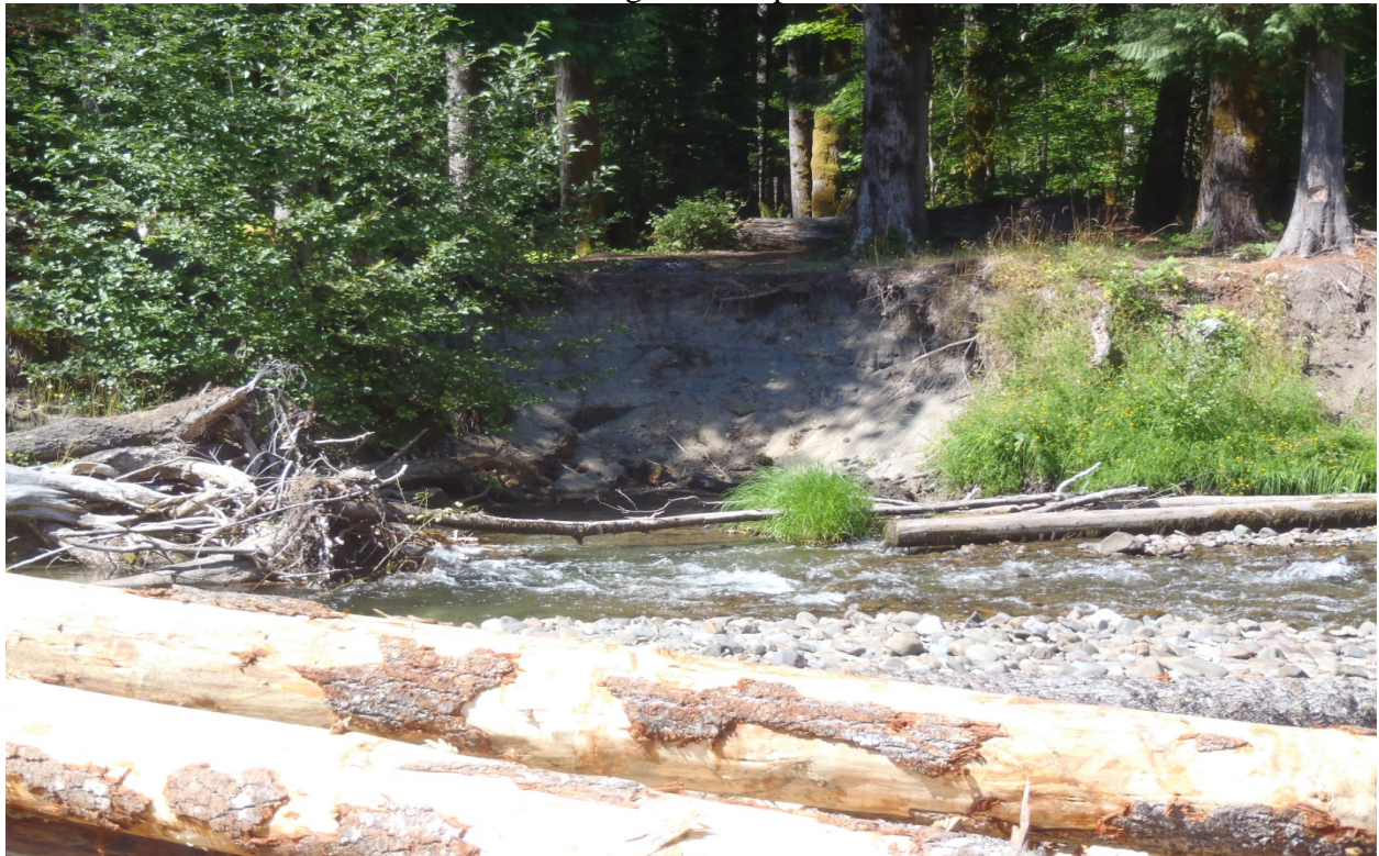
Looking across at eroding bank at ST#15 prior to construction
