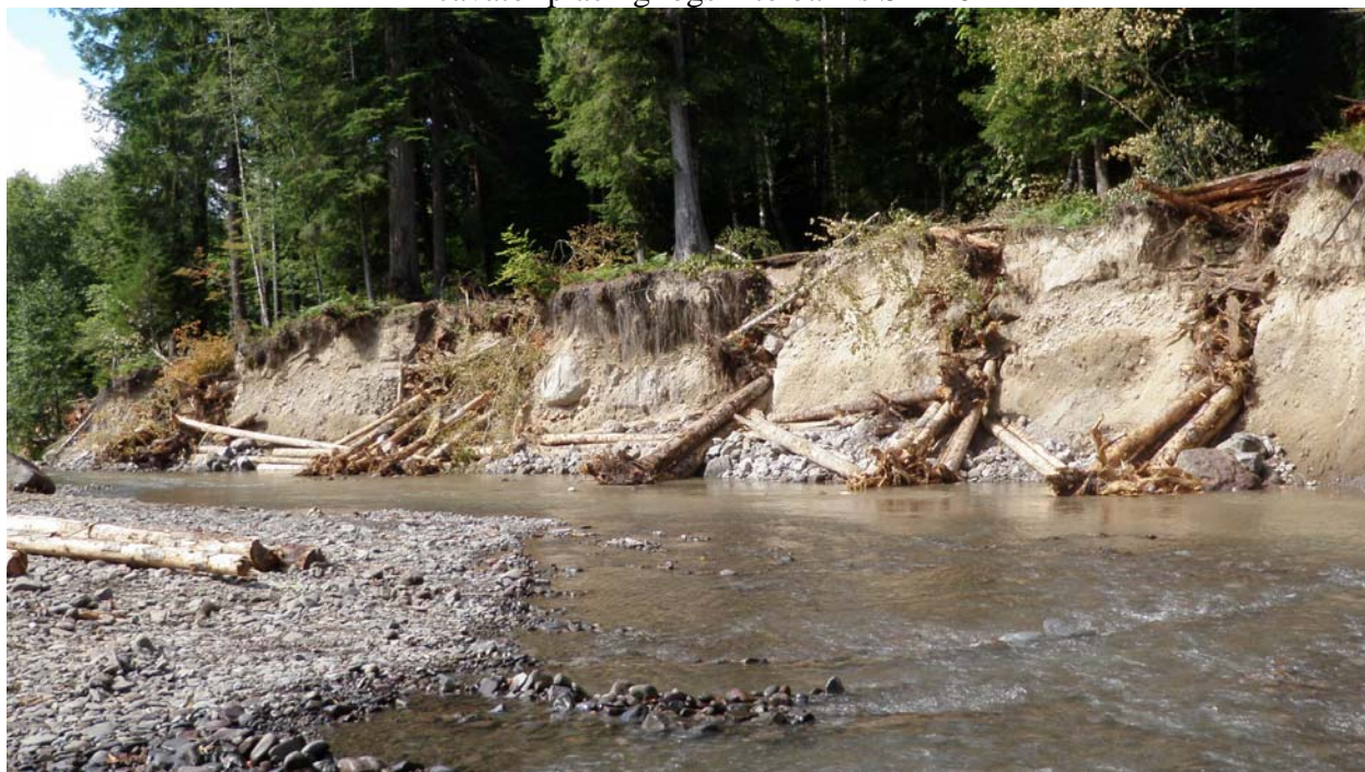
Completion of bank stabilization 87 logs was placed in eroding banks. Gravel bar on river left was shaved back 15-20 feet to help reduce flow on banks. ST#10
