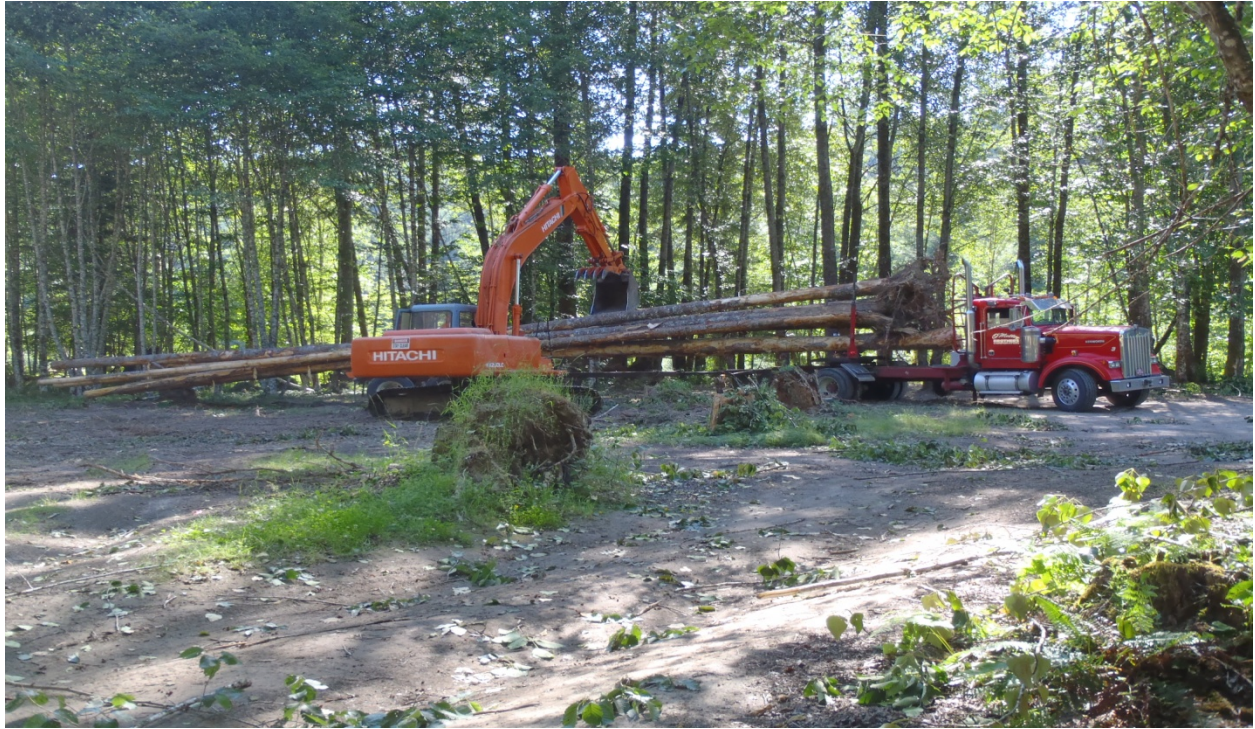
Unloading full lengths trees with rootwads
