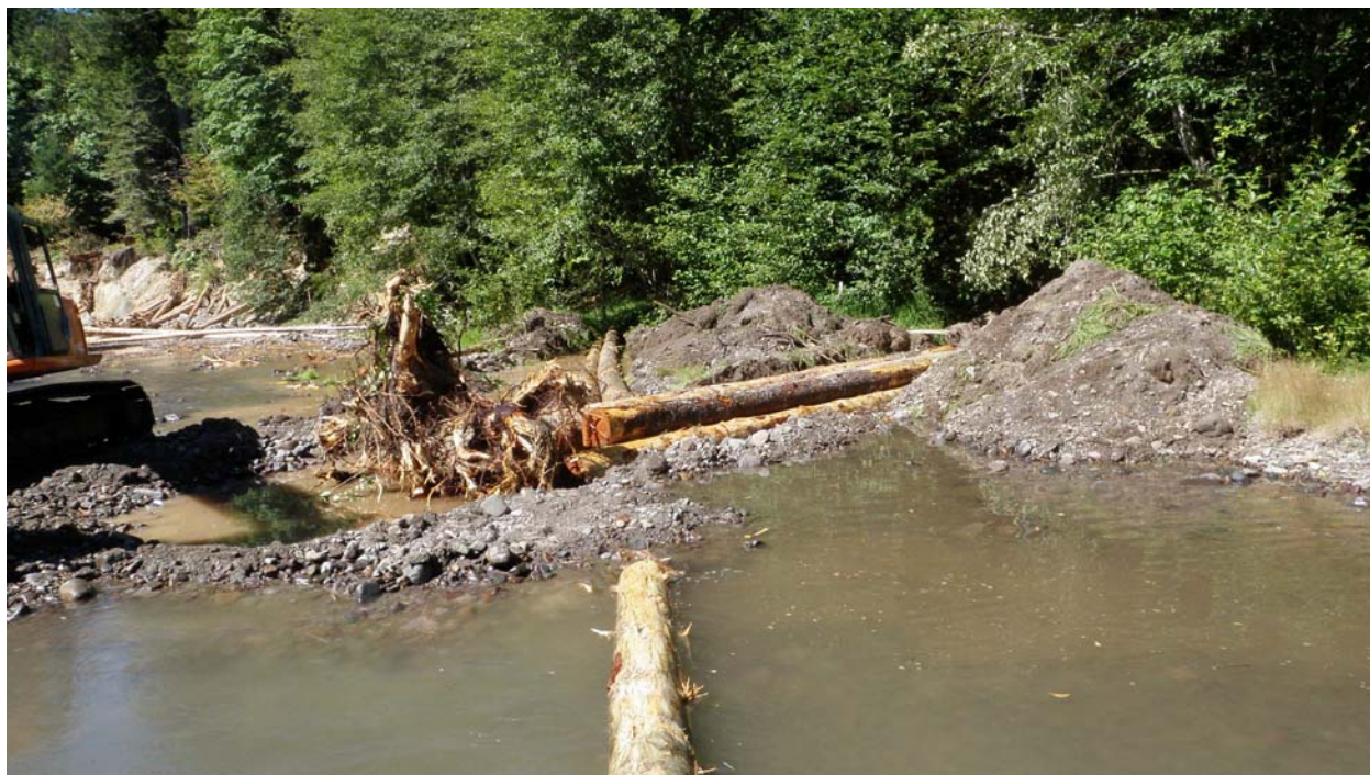
Start of the toe and anchor structure ST#12
