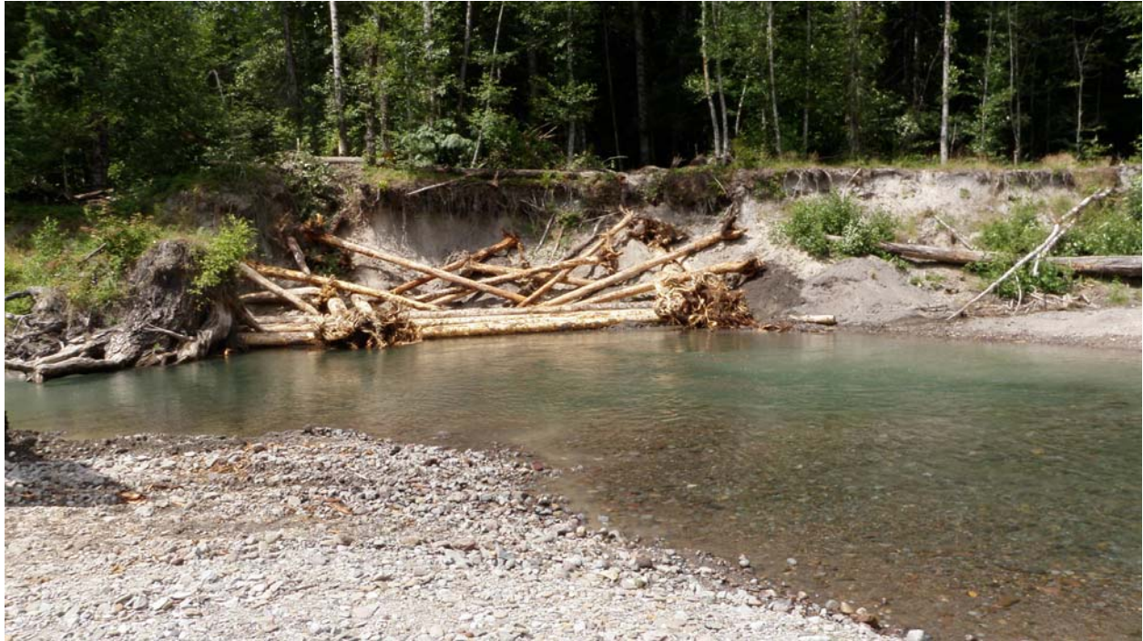
Looking down stream at bank stabilization structure 50 logs were placed in structure ST#2
