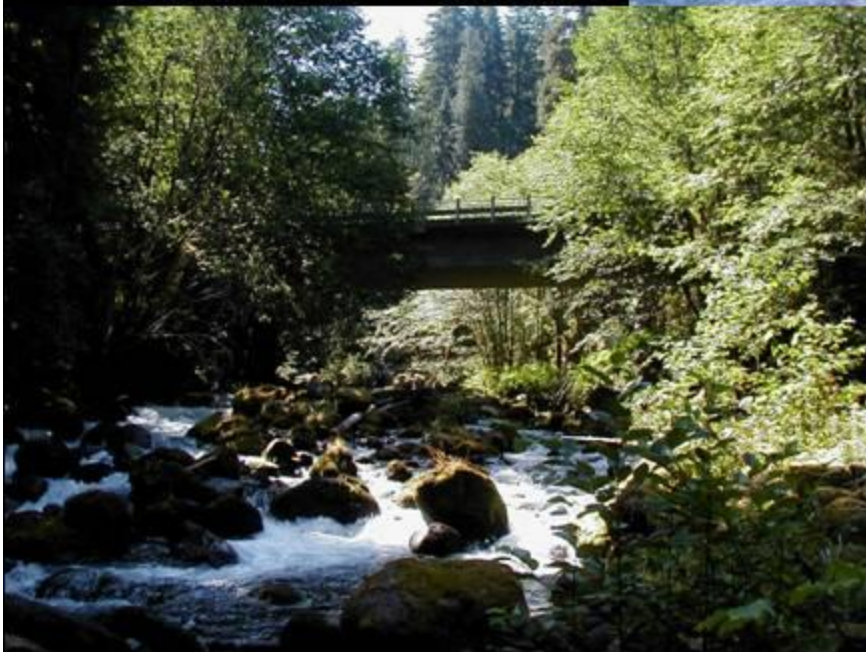
Photo 3 August 4, 2004 Reach 1 – SO4, F3 Looking up stream, Forest Road 90 bridge across Rush Creek.
