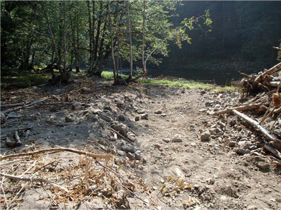
Photo 2. Lewis River side channel 5 project post implementation on 8/15/2017 (Photo B. Michaelis).
