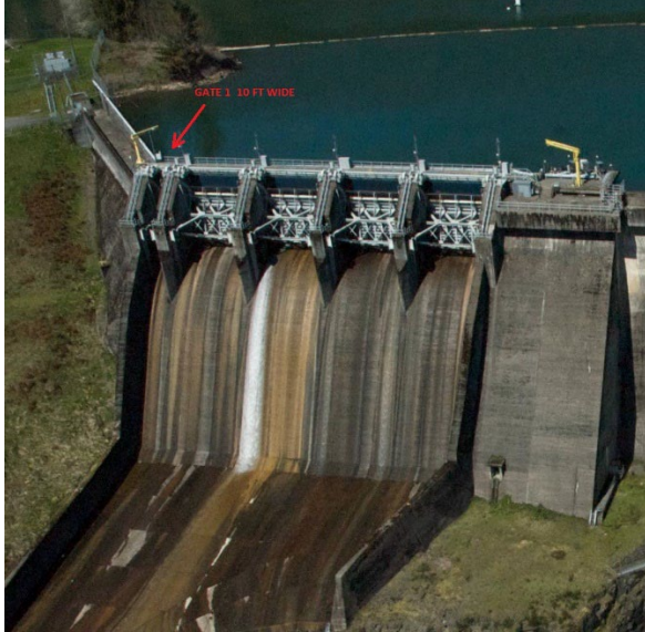
Photo of Merwin spillway, 10 ft wide gate on left
