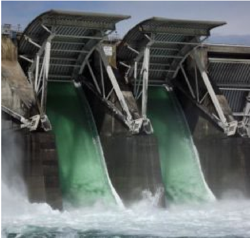
Retrofit spillway weirs in use, skimming surface flow, tainter gates raised out of the way
