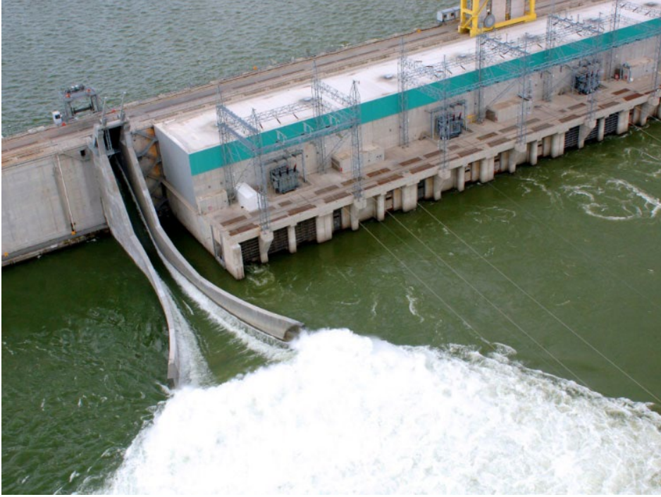
Skimming spillway gate with outfall chute built into dam
