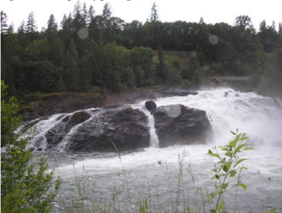
Figure 3. Yale spillway passing 4,100 cfs.
