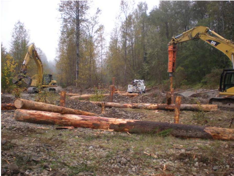
Figure 16. Installation of floodplain roughness LWD on the Cowlitz River (Inter-Fluve).
