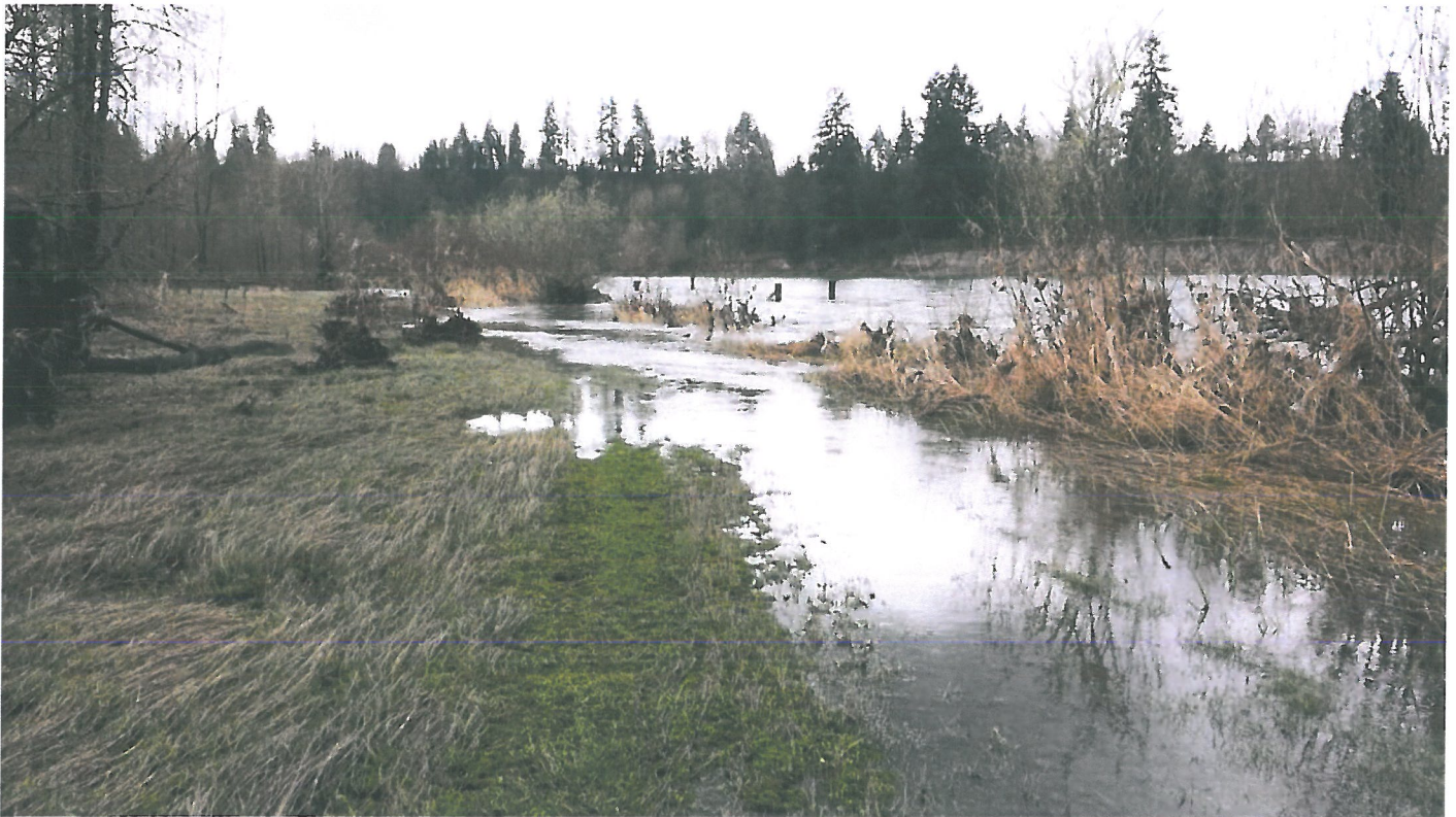
View downstream of proposed side channel during winter high water event. 2/3 of side channel flows in a ORV road
