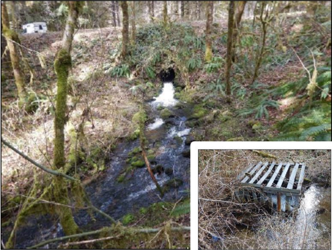
Figure 1. Culvert outlet (inlet bottom right) on FR-90. Note the high velocity, small size, perch, and lack of a jump pool.
