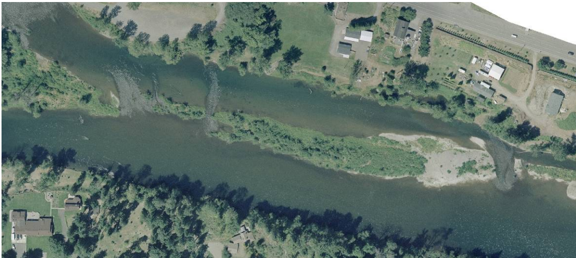
Aerial view of project site cross-over channels just upstream of bifurcation at upstream end of Eagle Island
