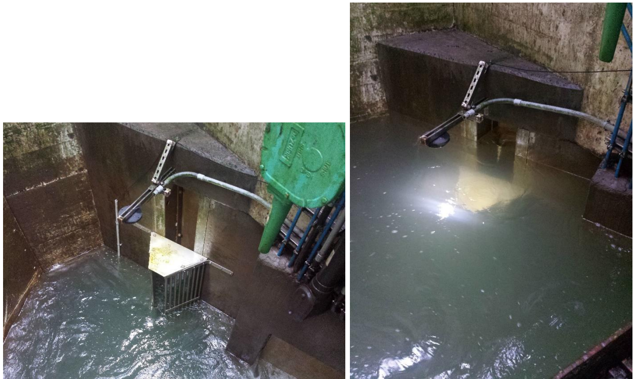
Figure 7. Photos of the entrance between Pool 1 and 2 within the trap ladder where the fyke was installed. The photos show the entrance during low (< 7,000 cfs; left photo) and high (~ 8,000 cfs; right photo) discharge when the water height was below and above the fyke height, respectively. Photo Credit: Chris Karchesky.
