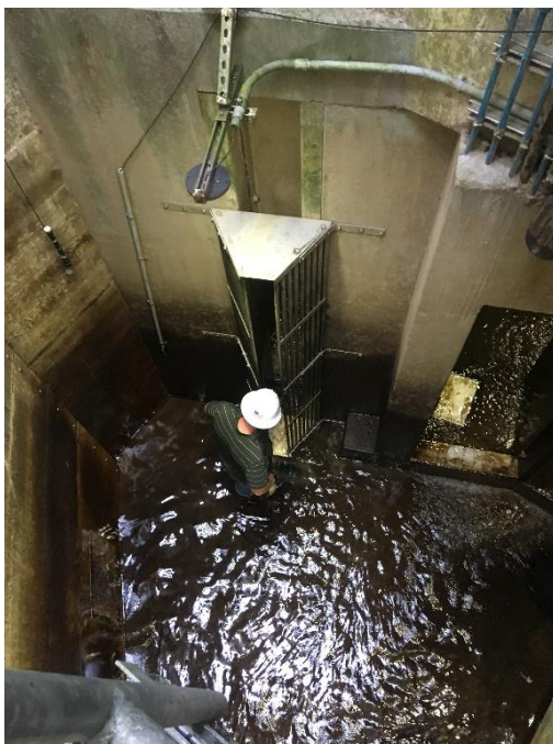
Figure 6. Photo of fyke installed at the entrance to Pool 2 within the trap area. Photo was taken looking down into Pool 2 from above during dewatering. Note there is a gap above fyke, where fish could potentially exit through. Photo Credit: L. Caldwell, August 22, 2017 during trap dewatering.
