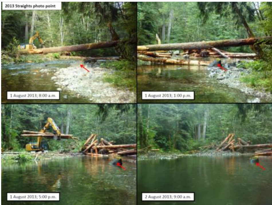
Figure 5. Photo sequence showing the elevation of the streambed with wood and boulders to reach the relict channel elevation after the removal of the push up berm. Still Creek, Mt Hood National Forest, Clackamas County, Oregon.
