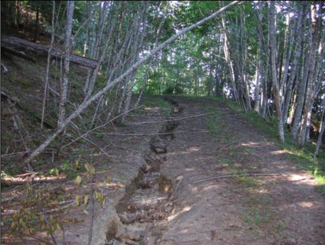
Surface erosion from blocked culvert on FR9300150.
