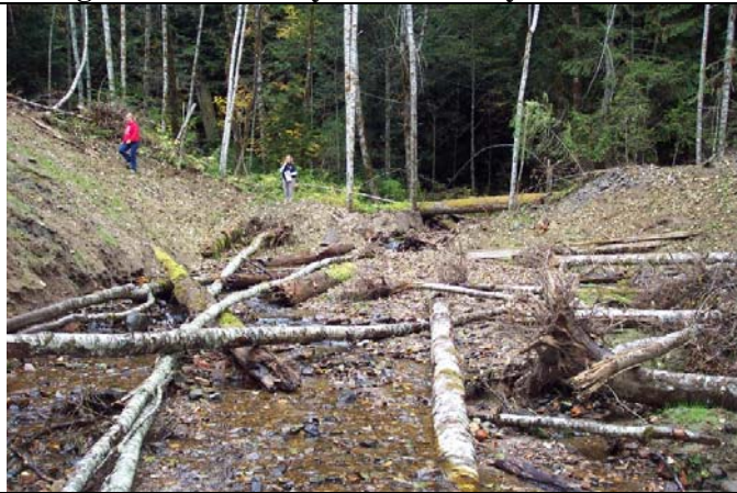
2008 Post – Project FR 8322700 Road Decommission – Road Fill Removed, Stream banks match adjacent natural slopes. Available large wood placed into stream and along stream bank, Trees still to be planted. Low gradient tributary to Muddy River.
