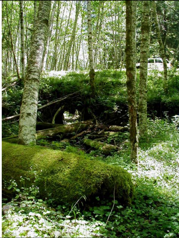
2006 Pre - Project FR 8322700 Road Decommission – Blocked Inlet, 1 foot drop at outlet. Low gradient tributary to the Muddy River.
