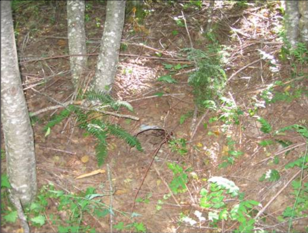
Blocked Culvert Inlet on FR9300150.
