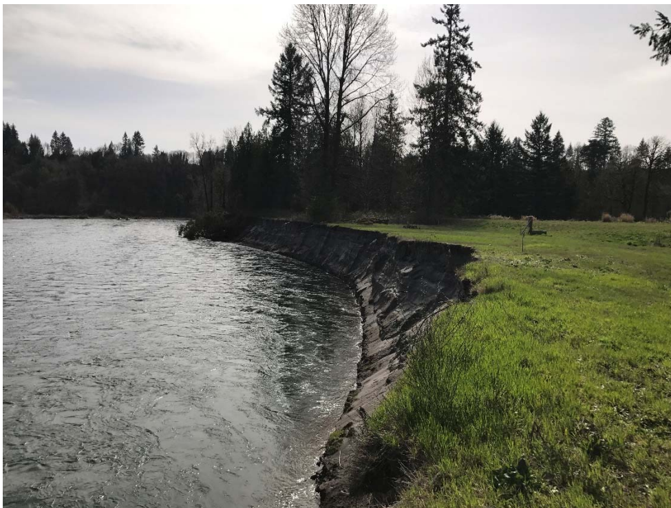
Photo by Cowlitz CD looking downstream along Anderson parcel showing bank erosion site and opportunity for riparian vegetation between river and the access road.
