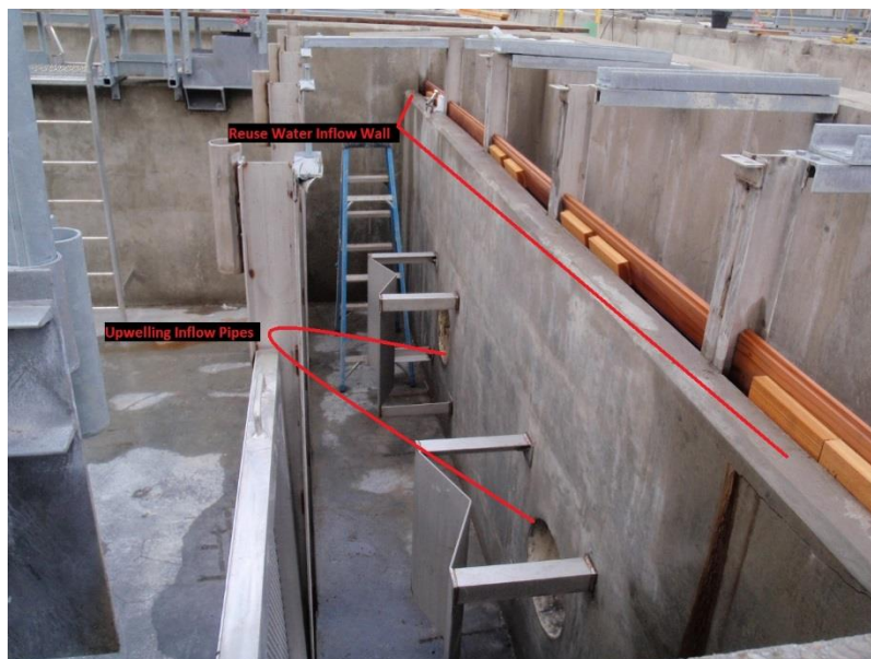
Figure 5. Location of the upwelling pipes and reuse water weir wall
