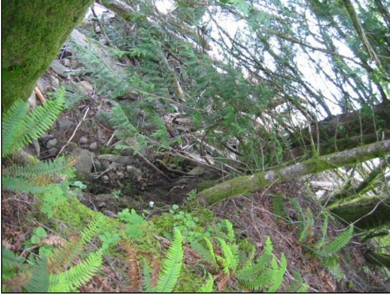
Figure 9: Slope Failure Area in Segment 2
