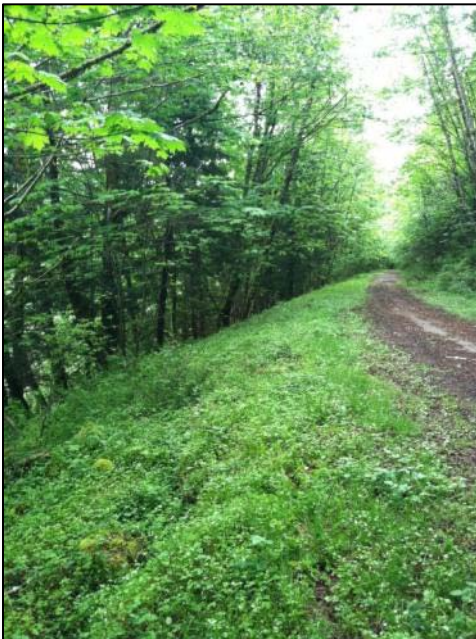
Figure 4: Slump of Downhill Fill Slope
