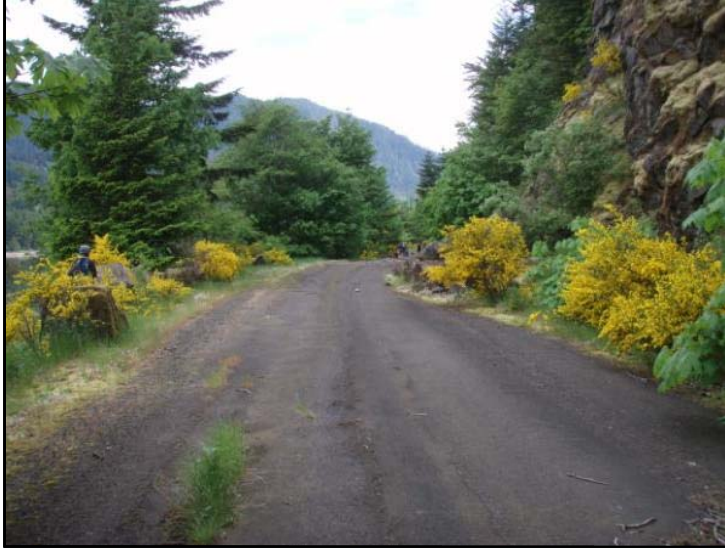
Figure 1: Slumped and Rutted Pavement Areas in Segment 2
