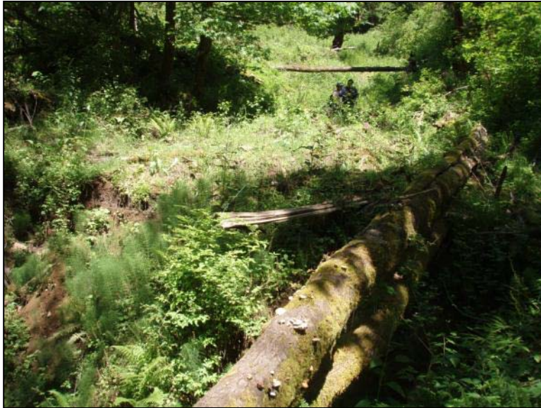
Figure 18: Slide Area in Segment 3
