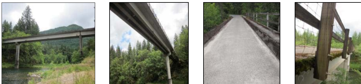
Figure 33: Lewis River Bridge (4 views)
