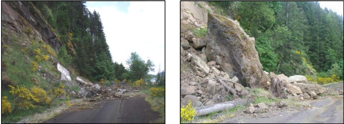
Figure 3: Examples of Larger Rockfalls (2 views)
