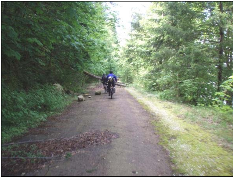
Figure 12: Pavement in Good Condition in Segment 2
