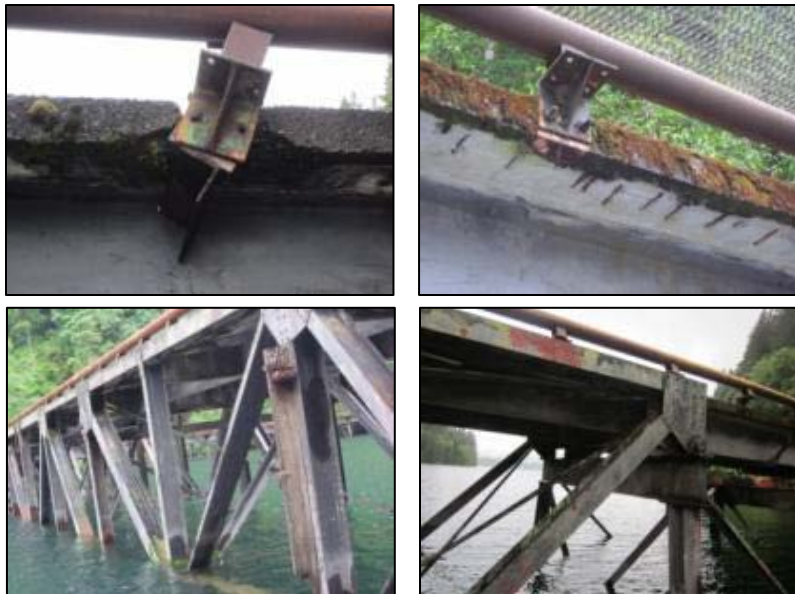
Figure 32: Siouxon Creek Bridge Defects (4 views)
