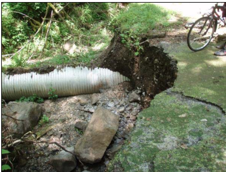
Figure 17: Slope Failure at Approximate Station 260+00
