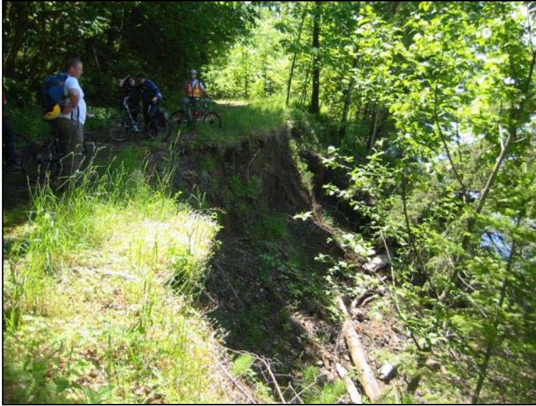
Figure 29: Eroded Cut Bank in Segment 4
