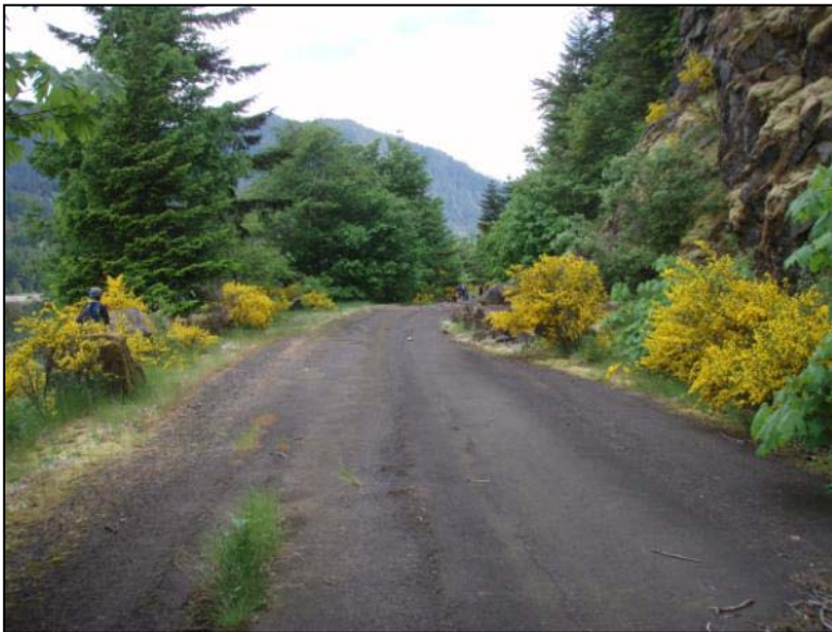
Figure 8: Slumped and Retted Pavement Area in Segment 2
