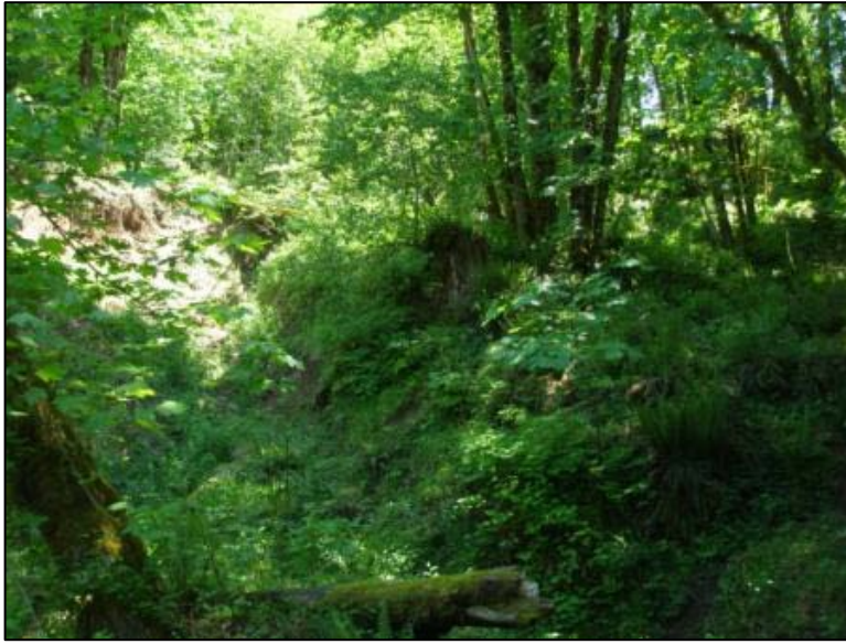
Figure 23: Upslope Headscarp and Landslide Debris
