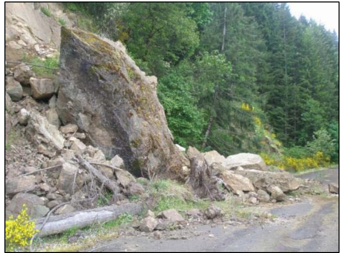
Figure 14: Example of Larger Rockfall Debris
