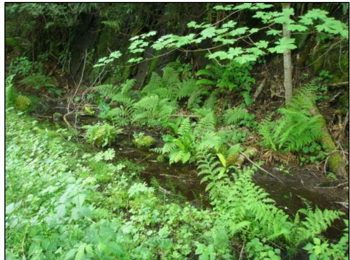
Figure 5: Poor Ditch Drainage Due to Blocked Culvert
