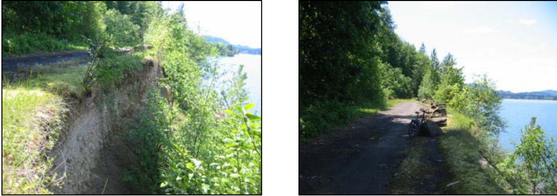
Figure 16: Slope Failure at Approximate Station 215+00 (2 views)
