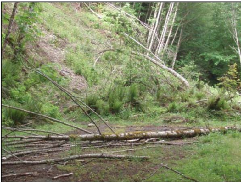
Figure 2: Slide Area in Segment 1
