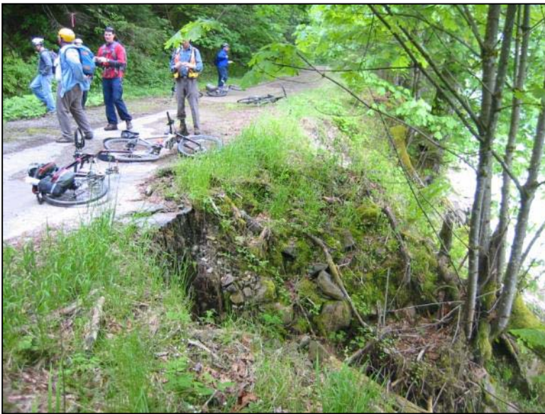
Figure 10: Bank Erosion Area in Segment 2
