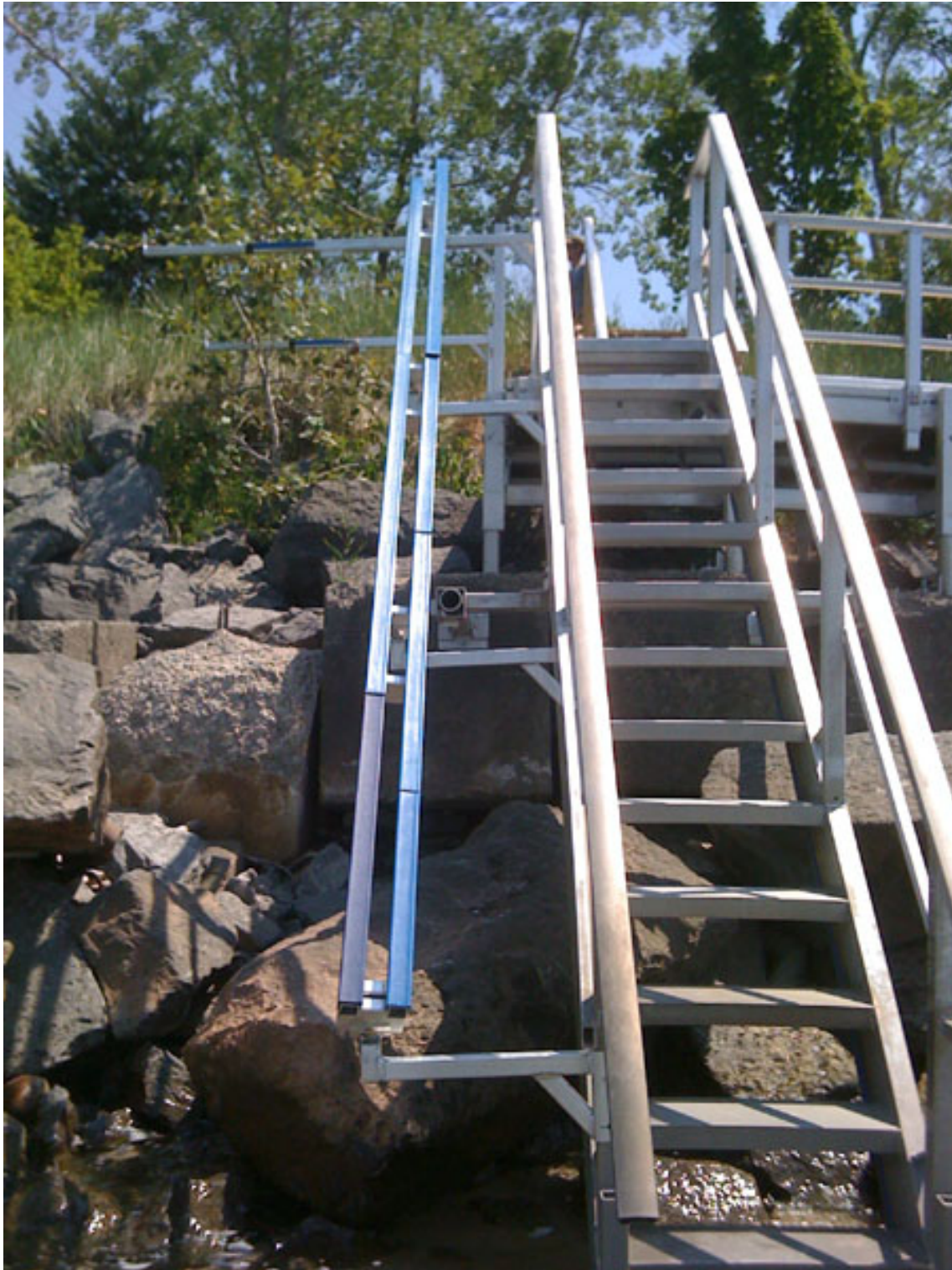
A light duty aluminum kayak rail attached to a dock stairway
