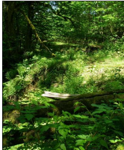
Figure 25: Debris and Road Undermining, Looking North
