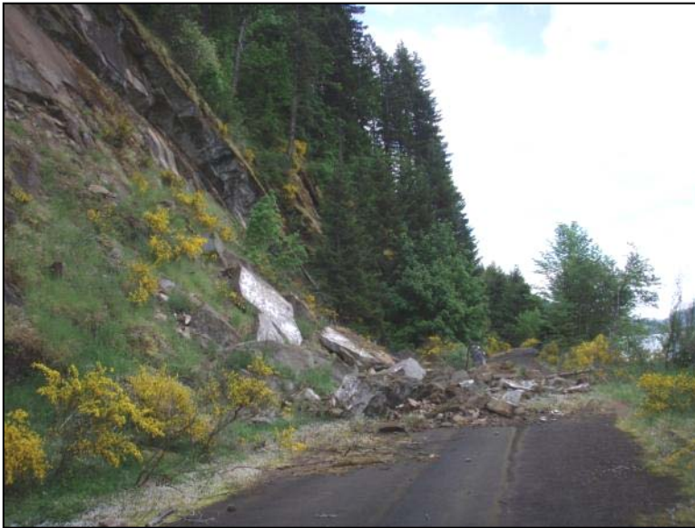
Figure 11: Rock Fall and Other Debris Area in Segment 2
