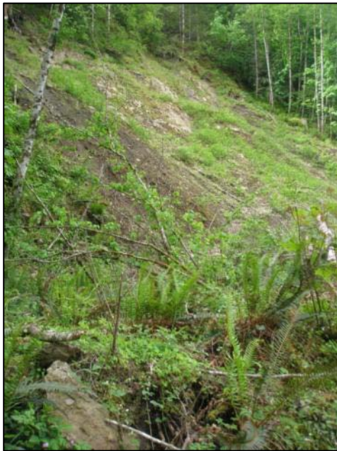
Figure 6: Slope Uphill of Landslide
