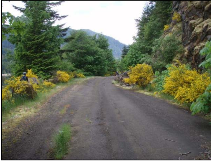
Figure 1: Slumped and Rutted Pavement Areas in Segment 2
