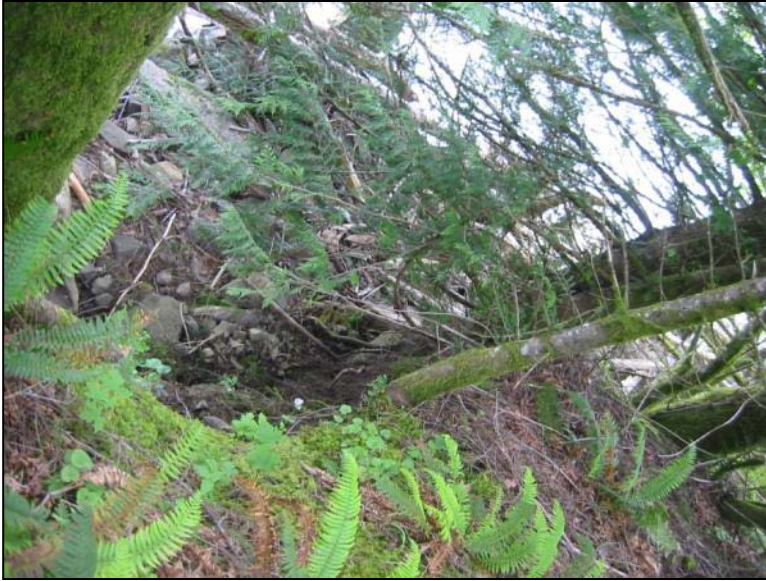
Figure 9: Slope Failure Area in Segment 2
