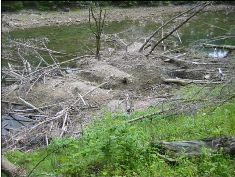
Figure 1: Toe Erosion in Segment 1
