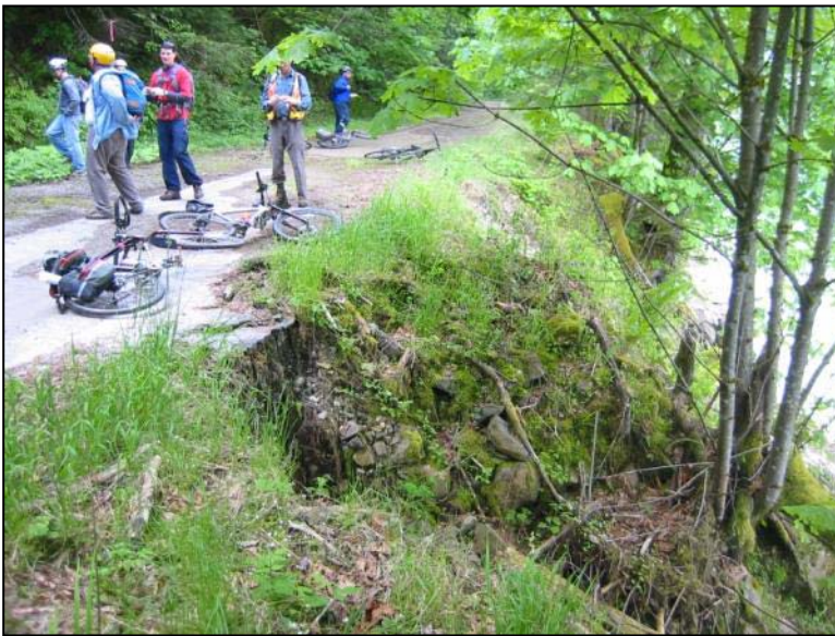
Figure 10: Bank Erosion Area in Segment 2
