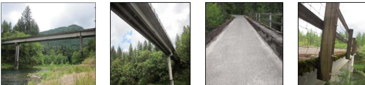
Figure 33: Lewis River Bridge (4 views)
