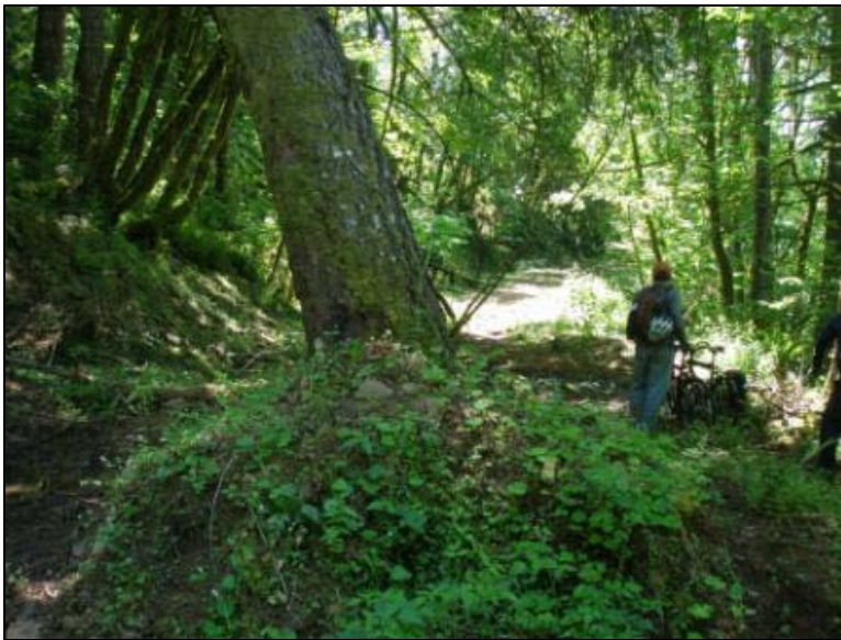
Figure 22: Tree and Landslide Debris in Middle of Road
