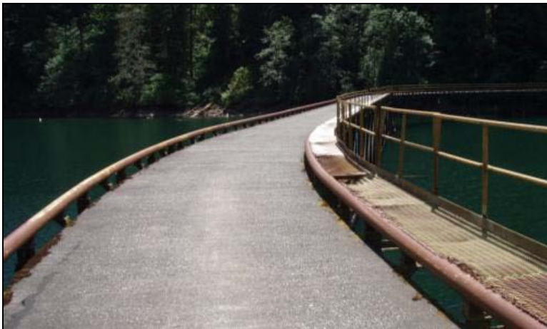
Figure 28: Siouxon Bridge at the Beginning of Segment 4
