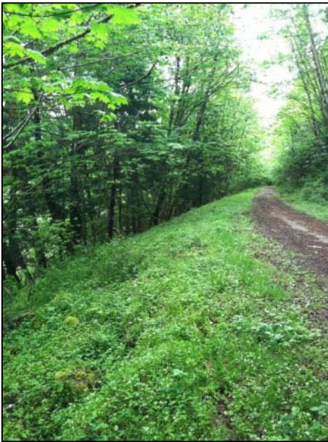
Figure 4: Slump of Downhill Fill Slope
