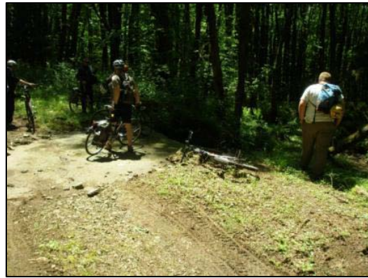
Figure 27: Debris Over Road Caused by Plugged Culvert
