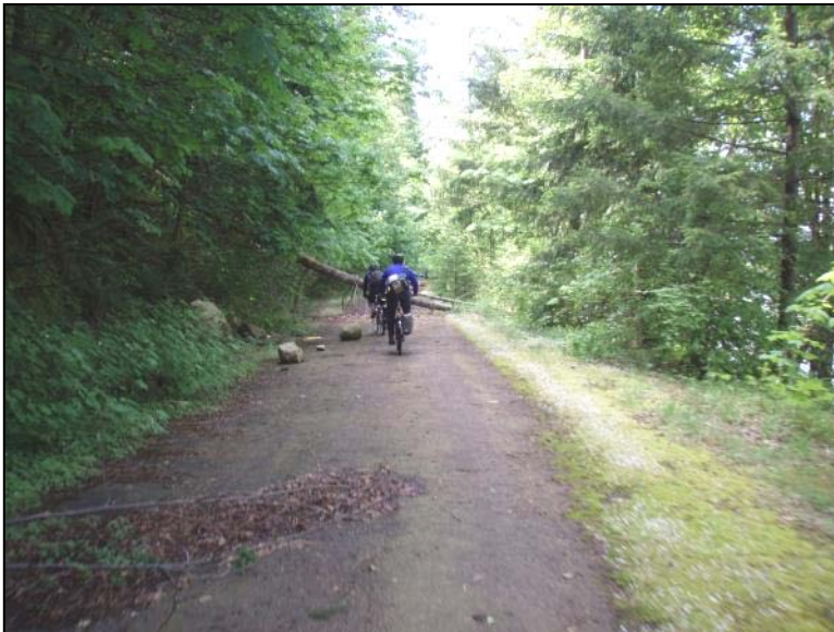
Figure 12: Pavement in Good Condition in Segment 2
