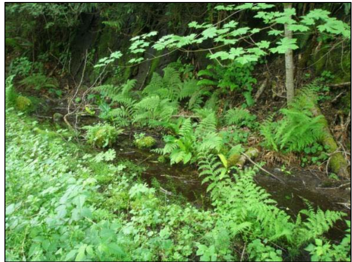
Figure 5: Poor Ditch Drainage Due to Blocked Culvert
