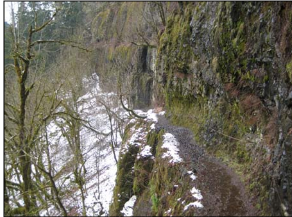
Example of a trail bench blasted from a basalt cliff near Bonneville Dam in Oregon.
