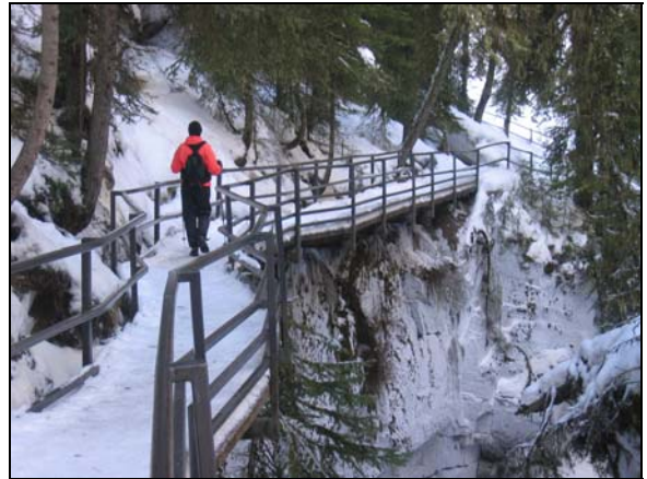
Examples of a cantilevered trail structure. (Image courtesy of Trail Dynamics)
