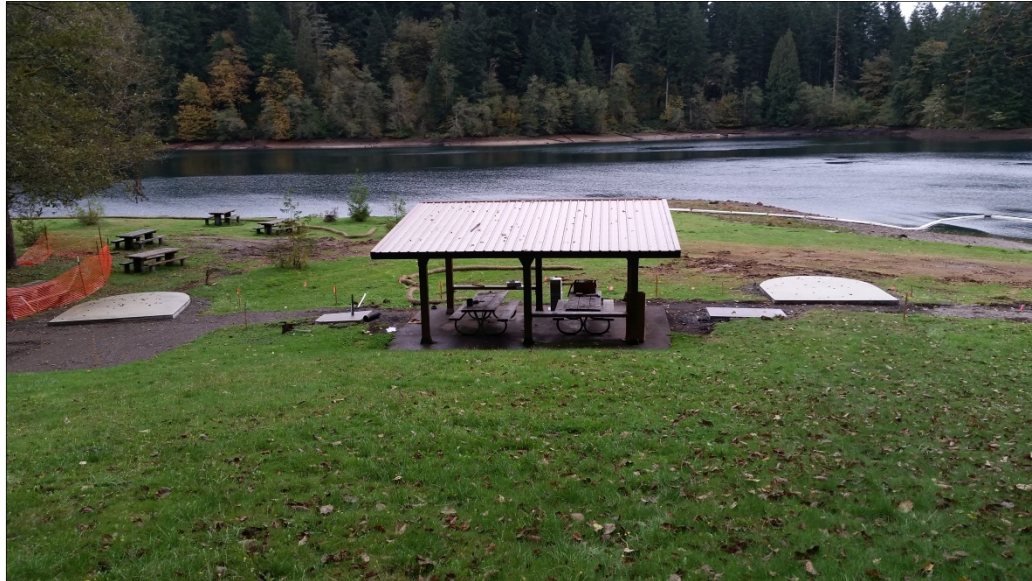
Speelyai Bay Park Accessibility Upgrades
