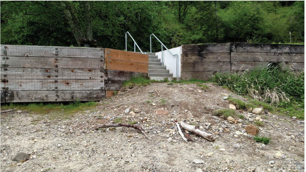
EXISTING WOOD BULKHEAD AND STAIRS
