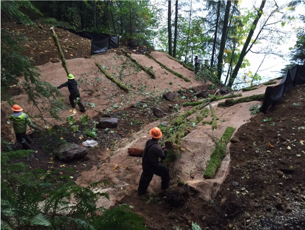
Figure 13. Culvert removal and soil stabilization along IP road in 2015.
