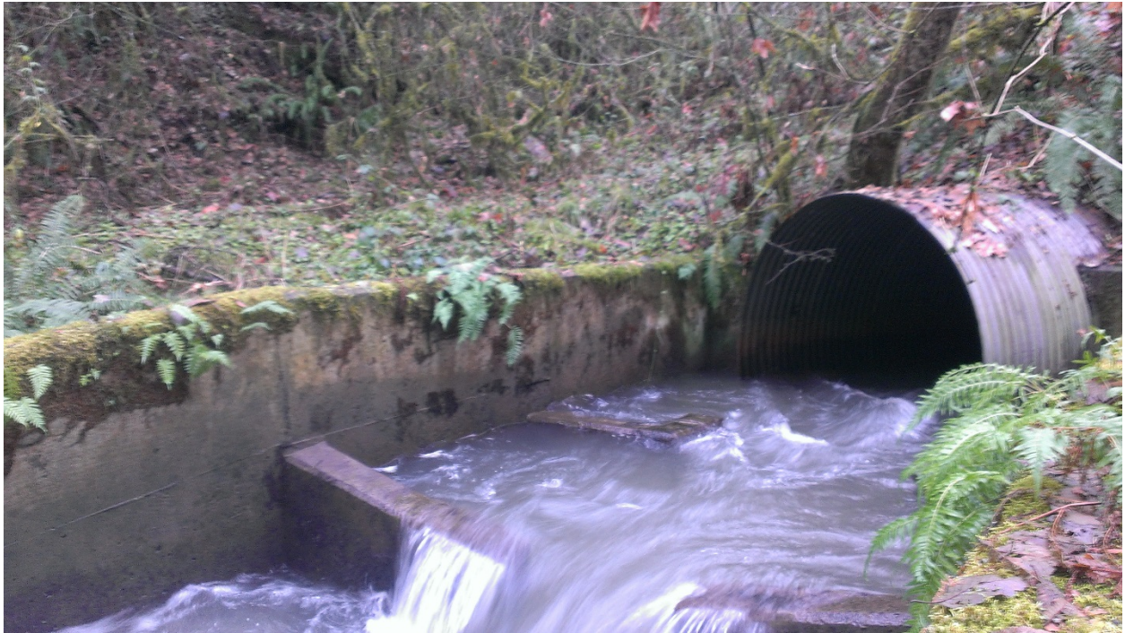
Photo 2: Riley Creek at Johnson Creek Rd.; a pipe culvert that does not fit the project description; but does have a fishway.
