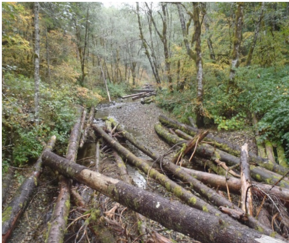
Photo 3: Gravel retention from habitat structure.
