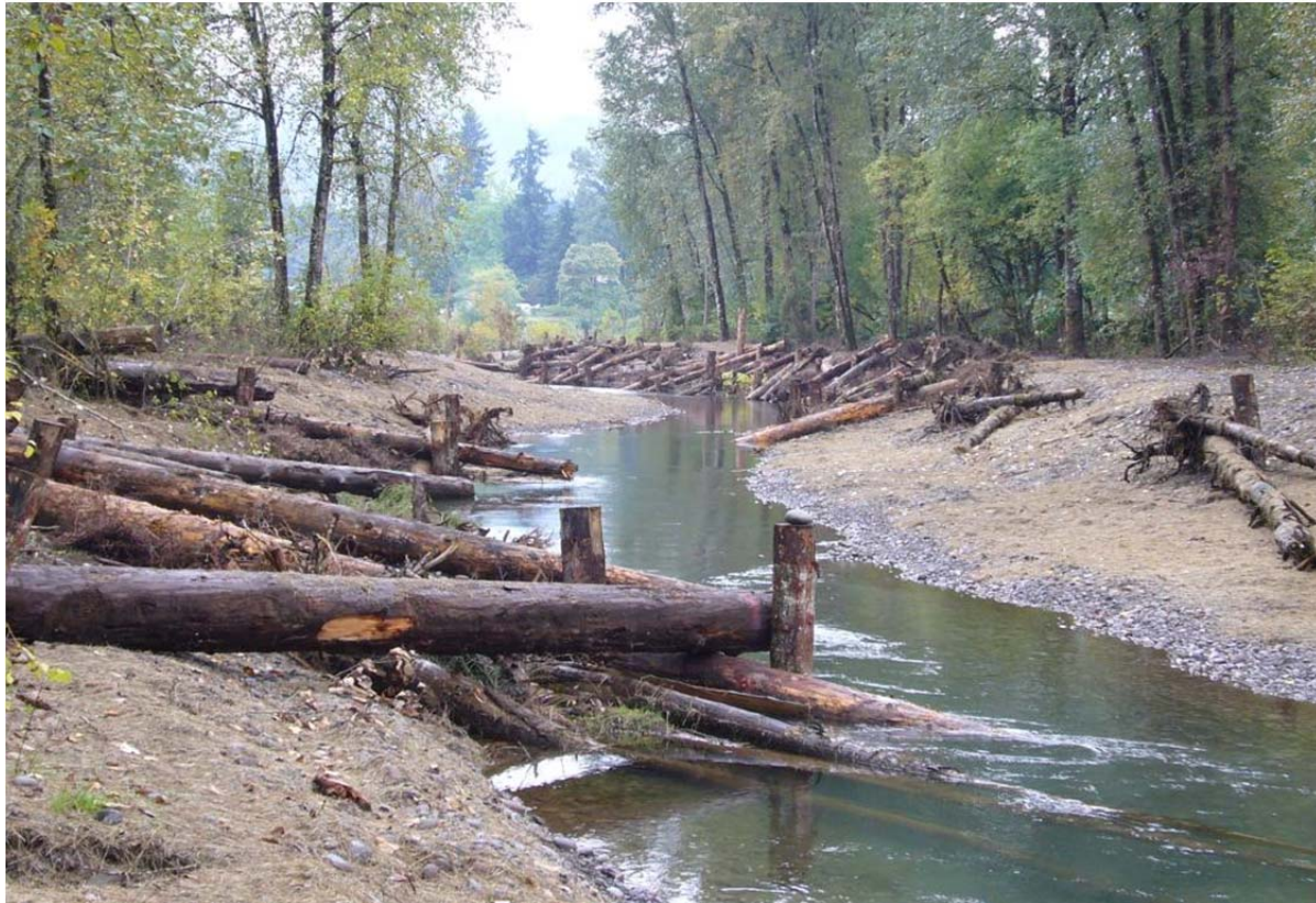
Photo 1: LWD in the side channel shortly after construction in 2011.
