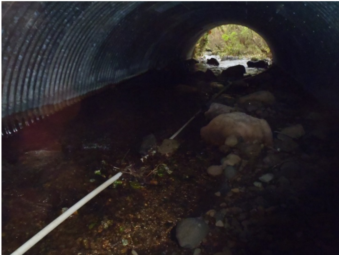
Photo 2: Looking upstream at natural channel conditions within the replacement culvert.
