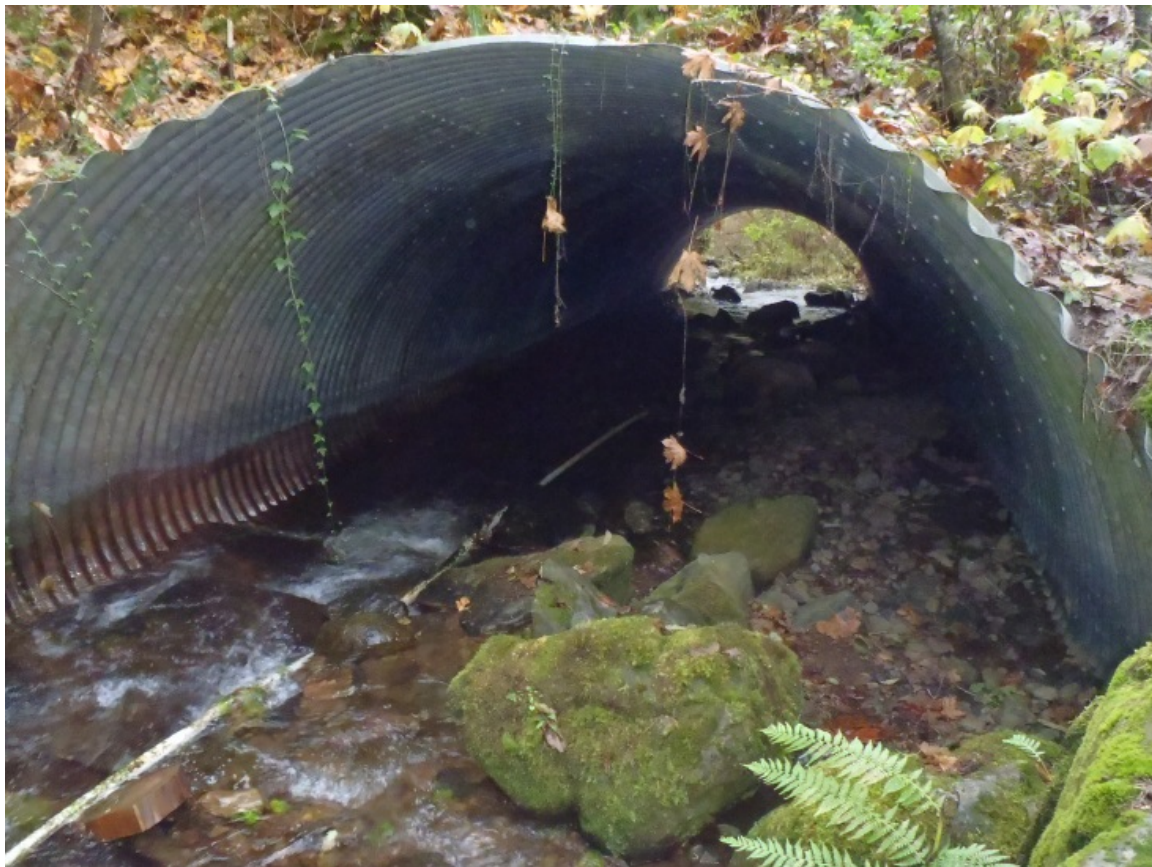
Photo 1: Natural channel conditions exist in this culvert on a tributary to Cedar Creek.
