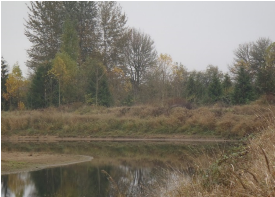
Photo 2: The bank has been stabilized with riparian plantings.
