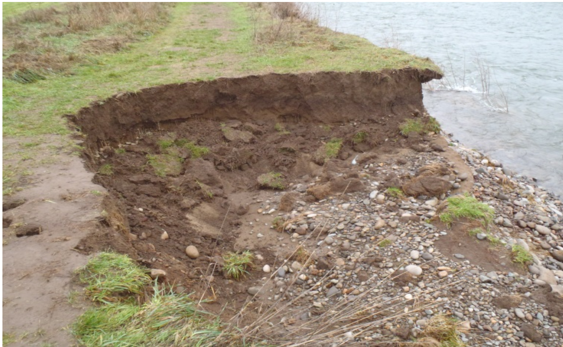
Photo 2: Erosion in the uncompleted portion of the project.
