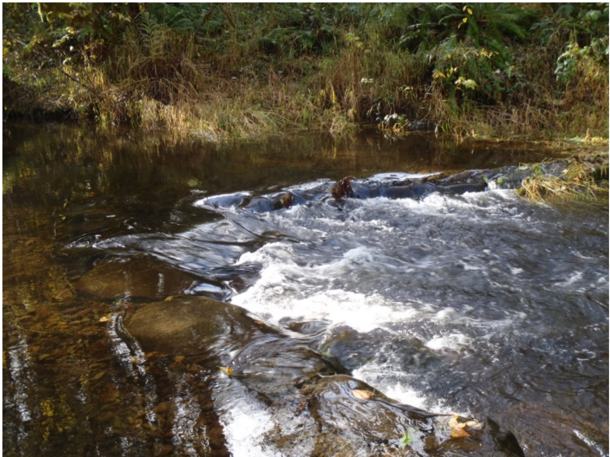
Photo 1: Rock vane and spawning gravel in Cedar Creek
