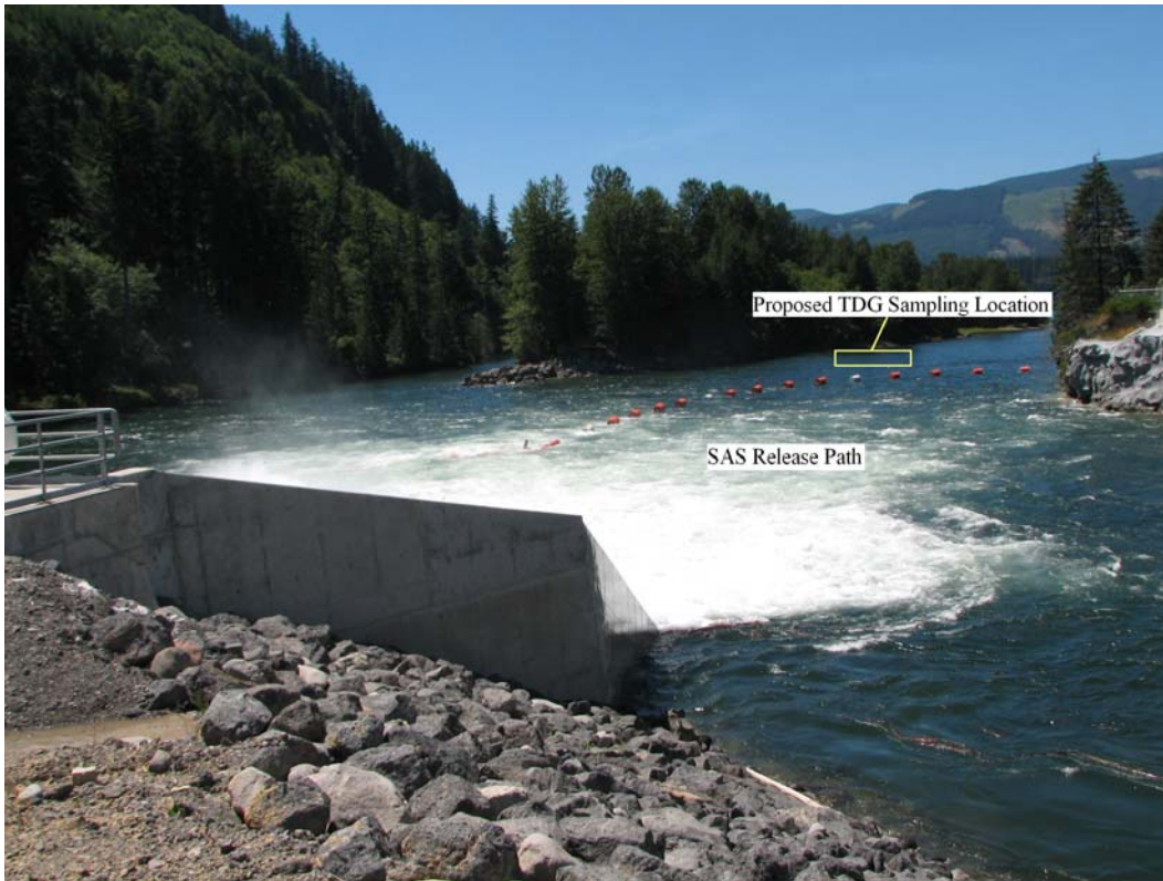
Photo 1. Photograph of the SAS during operation.
