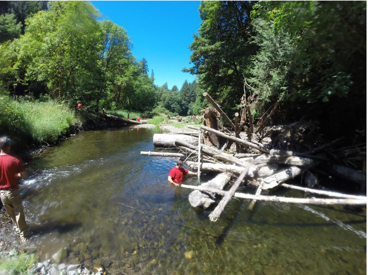
Checking post project pool depth
