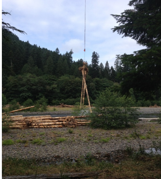
LWM being dropped by helicopter
