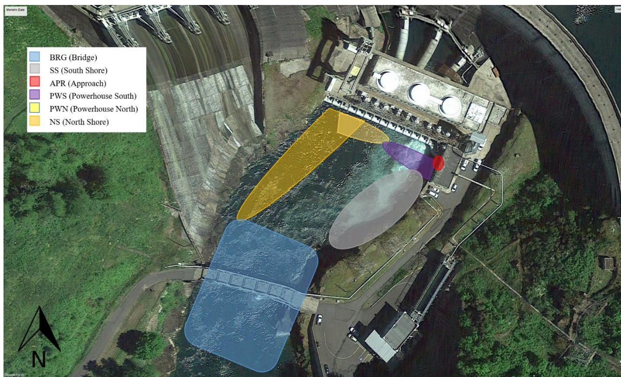
Figure 5. Locations of intended detection regions for six radio receivers located from the bridge upstream and into the fish passage facilities at Merwin Dam.
