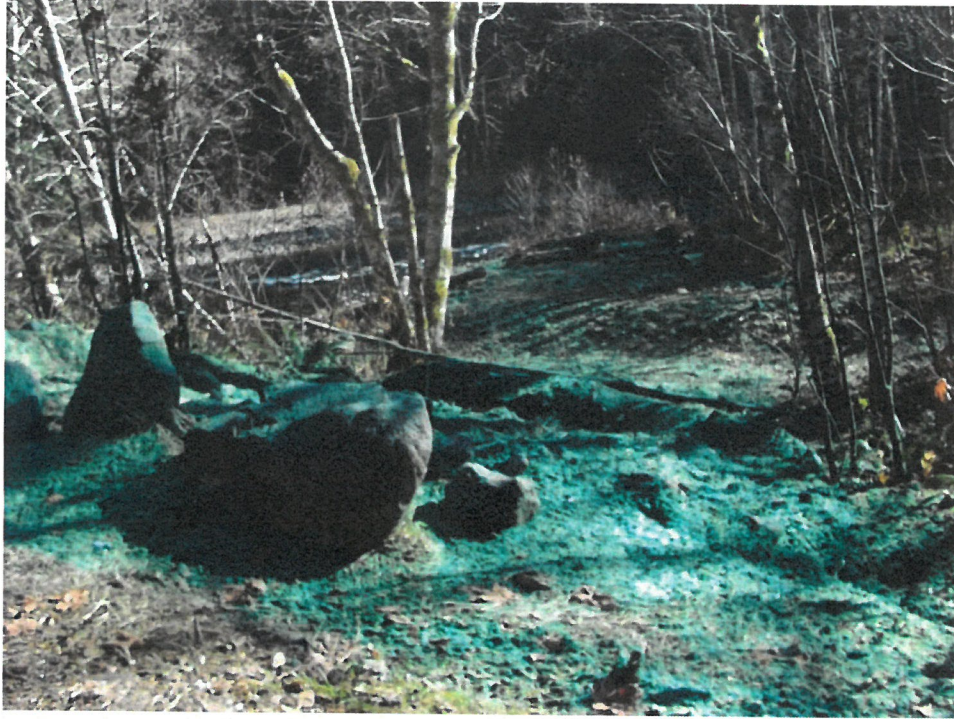
9. Clear Creek intake location restored, hydroseeded and planted with native plantings (November 5, 2019).
