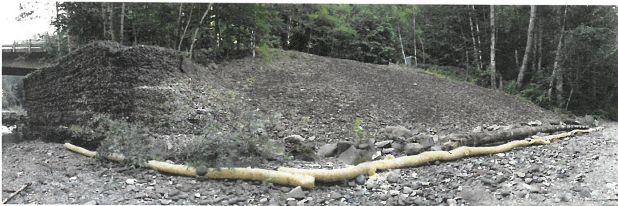
6. Crab Creek post-decommissioning (September 2019). Note final erosion control (jute matting) was installed the day after this photo was taken.
