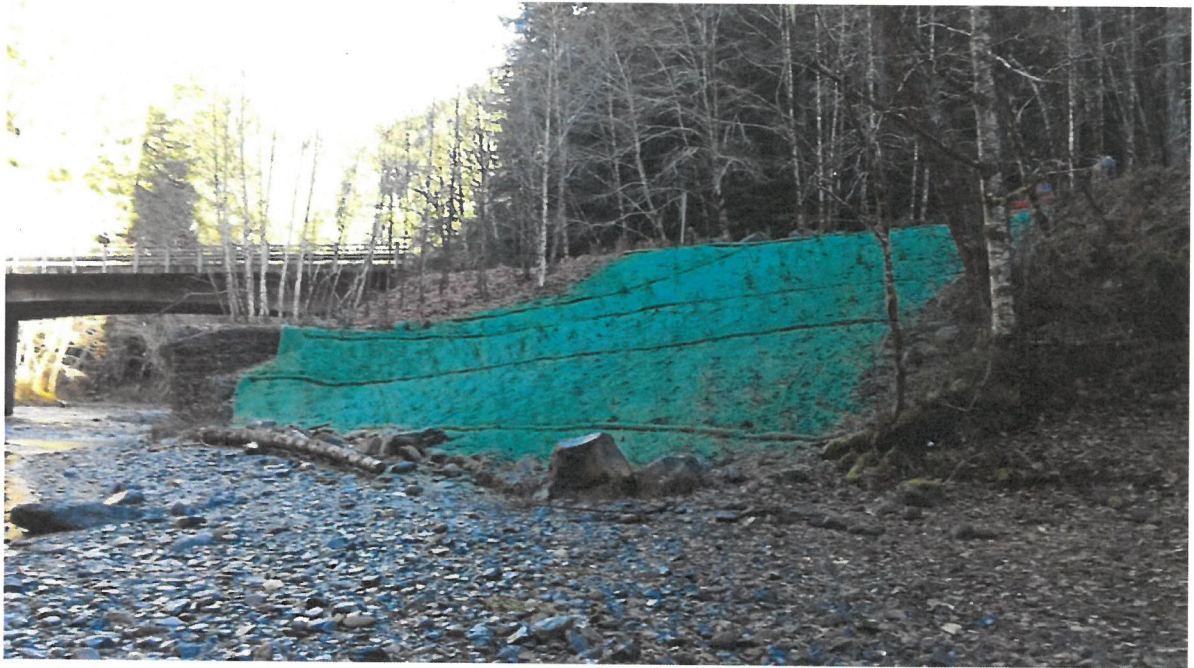
7. Crab Creek post-decommissioning. Note the erosion control, jute matting and native plantings (November 5, 2019)
