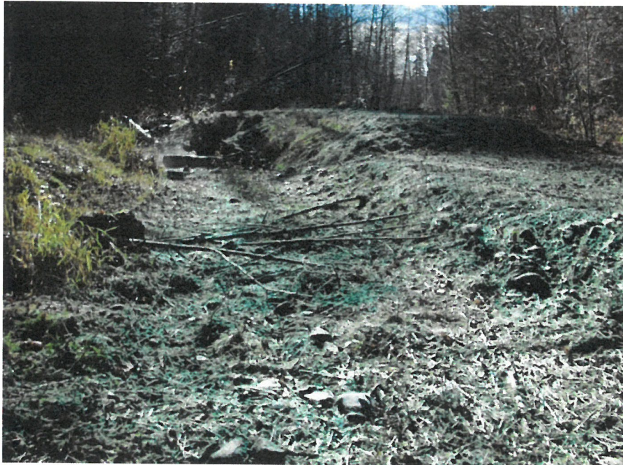
10. Clear Creek post-decommissioning. Note the constructed berm has been breached to re-connect Clear Creek to the floodplain (November 5, 2019).
