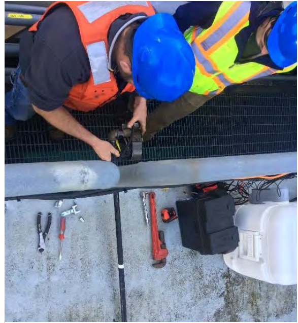
Appendix Figure A.2. Deployment of a collection channel hydrophone and mount, showing location behind the dewatering screens on the collection channel platform.
