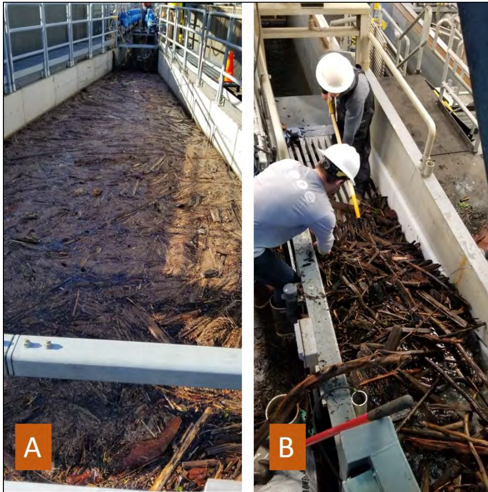
Figure 3.5-3. Woody debris accumulated within the fish passage channel (A), and on the sorting bars (B) within the Swift FSC in 2020.
