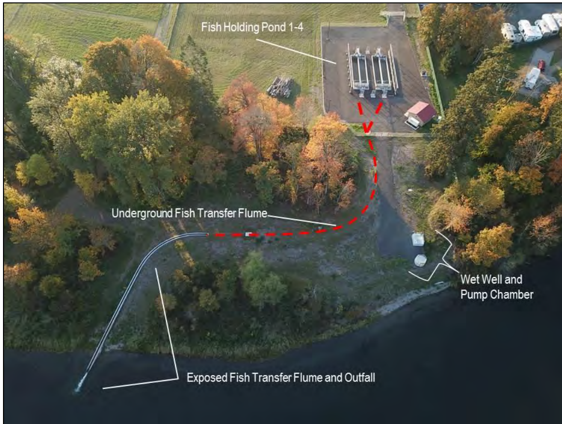
Figure 2.3-1. Aerial photo of the Woodland Release Ponds and associated infrastructure near Woodland, WA.
