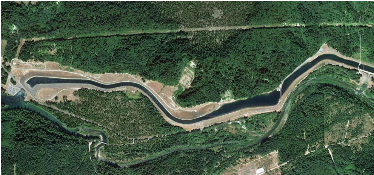
Figure 3.2-1. Project Works Management Unit (Google Earth, August, 2012).
