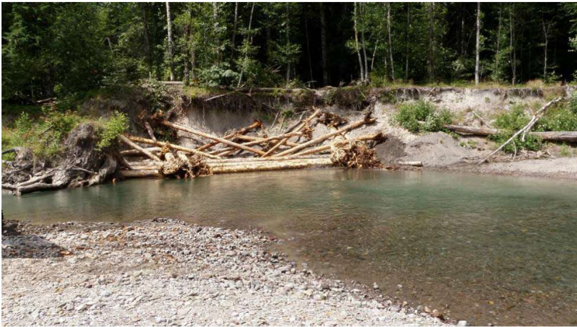
Figure 5. Example of a bank protection structure constructed on Clear Creek, 2010. Approximately 50 trees were used in this structure.
