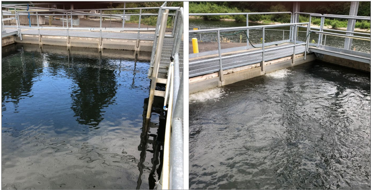
Figure 2. Illustration of flow changes with installation of flow boxes in raceway 13-4. Left picture illustrates upwelling inflow in raceway 13-1 (control); Right picture illustrates flow pattern with flow boxes installed in raceway 13-4.
