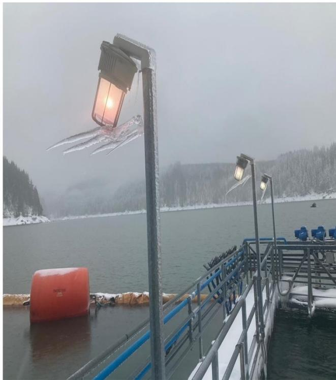
**Figure 2.1-2. Ice formation on the NTS and leading edge of the Swift FSC during the February 11, 2021 inclement weather conditions.**
