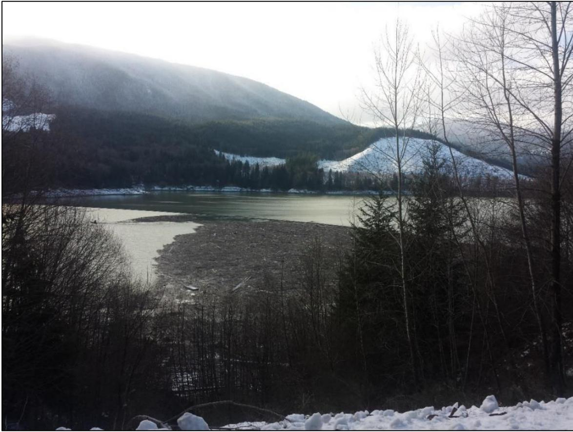
**Figure 3.5-2. Woody debris accumulated behind the upper debris boom located near the head of Swift Reservoir.**
