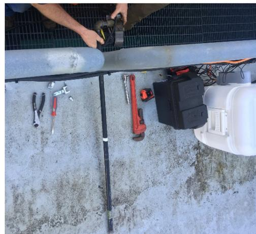
**Appendix Figure A.2.** Deployment of a collection channel hydrophone and mount, showing location behind the dewatering screens on the collection channel platform.
