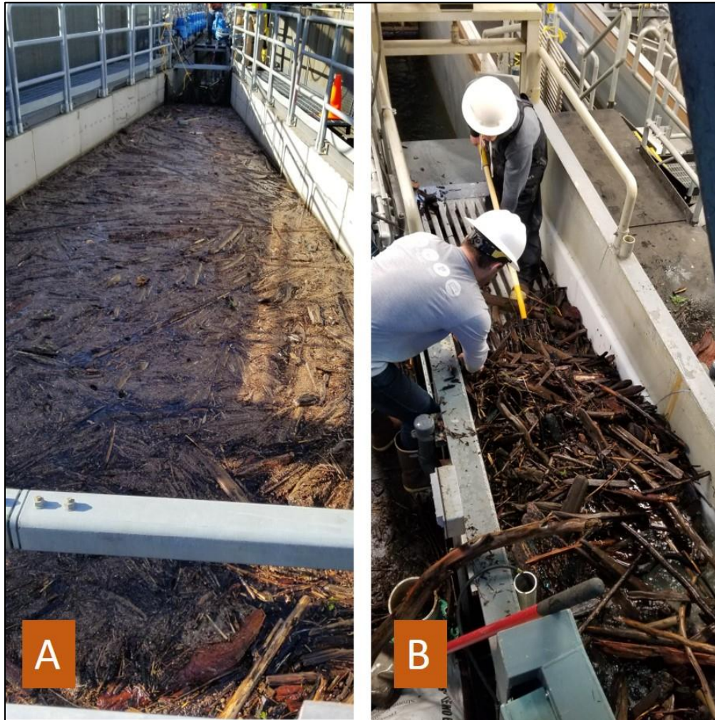
Figure 3.5-3. Example of woody debris accumulated within the fish passage channel (A), and on the sorting bars (B) within the Swift FSC.
