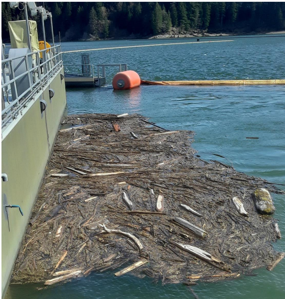
Figure 2.1-2. The debris weir, located on the south side of the NTS, allows debris to bypass the FSC during periods of heavy debris loading.
