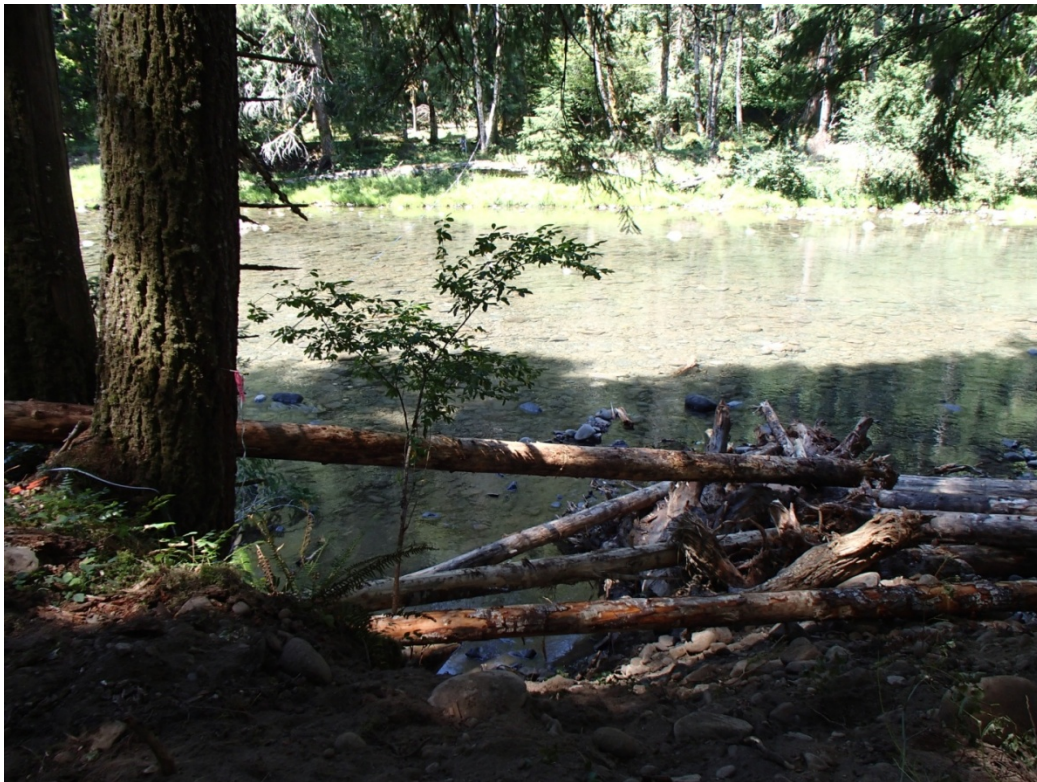
Structure 3 - Looking left bank to right bank
