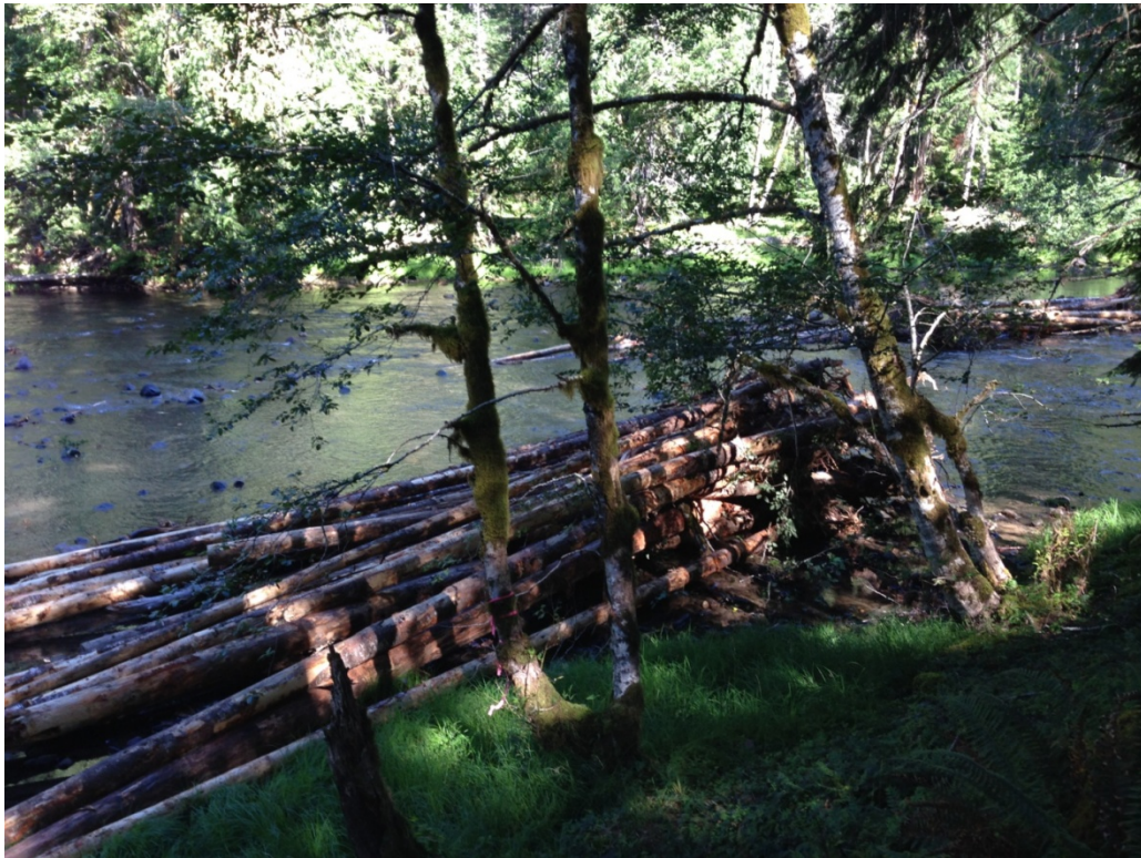
Logs placed into piles in the river before installation
