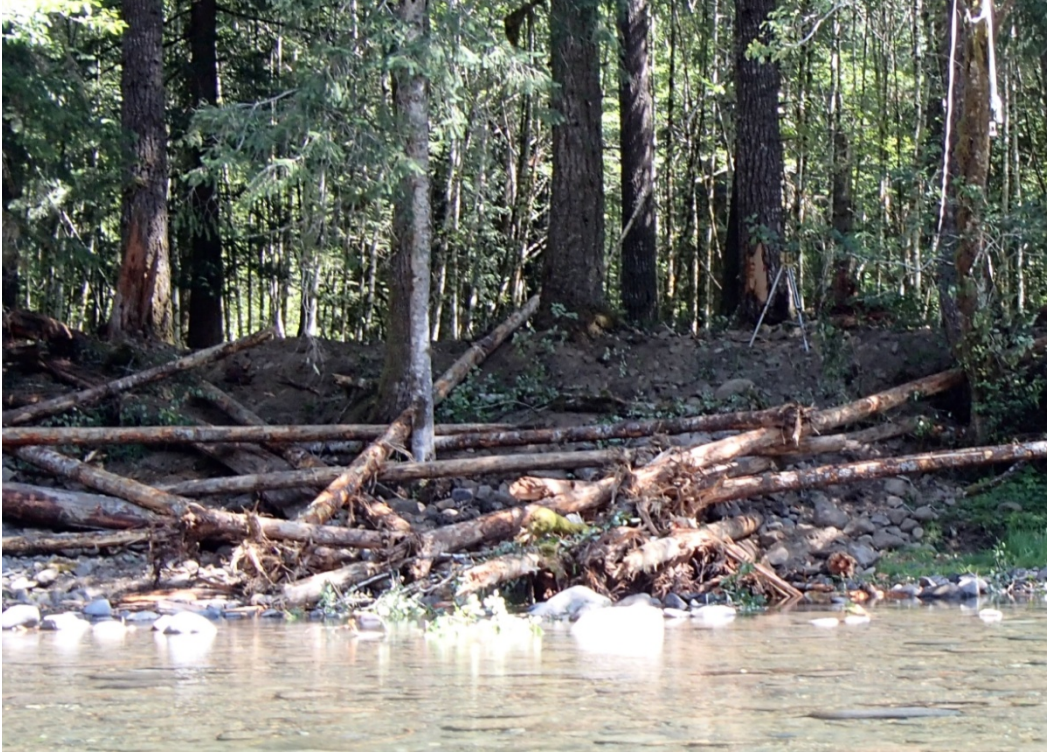
Structure 4 - Looking right bank to left bank
