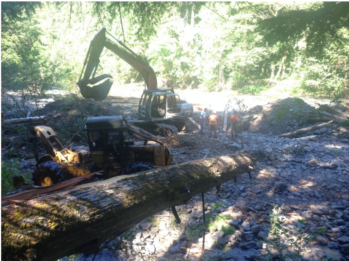
Skidder placing logs, excavator building apex log jam
