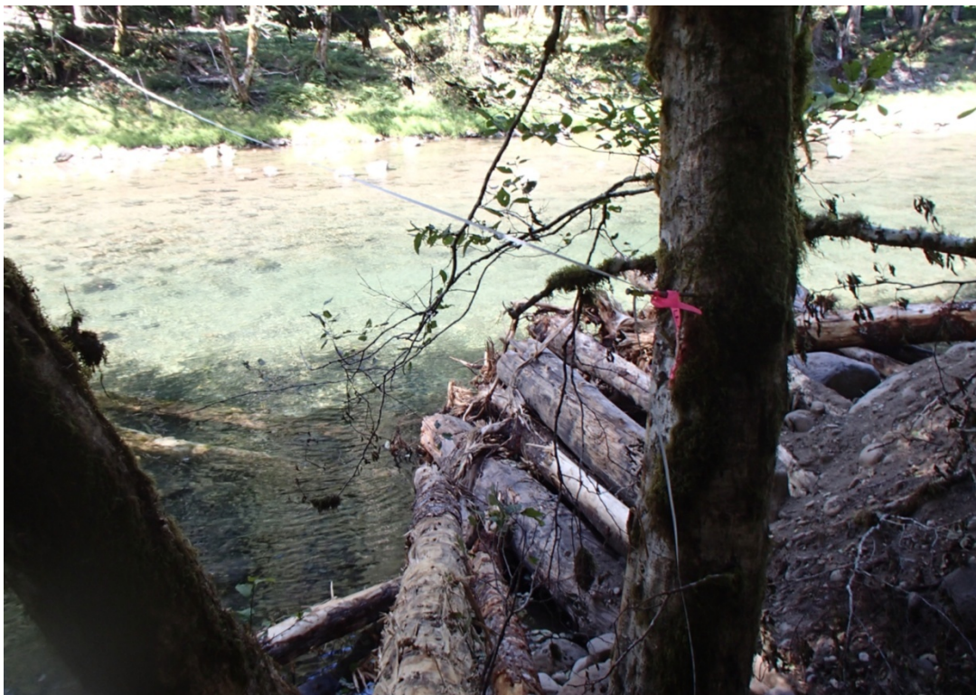
Structure 7 - Looking left bank to right bank
