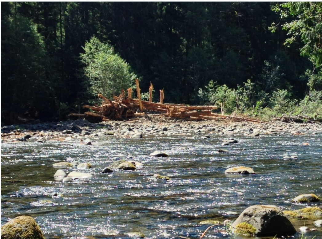
Non-numbered structure apex log jam on rocky island in center of channel, below other structures
