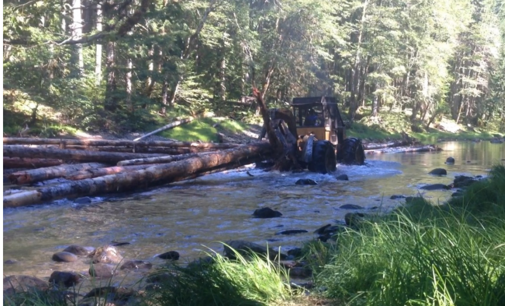
LWM being hauled into place on the North Fork Lewis River
