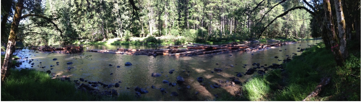
Logs placed into piles in the river before installation
