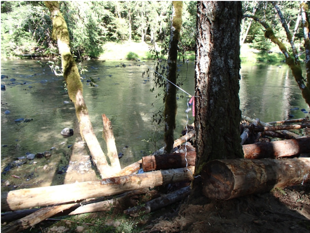
Structure 1 - Looking left bank to right bank
