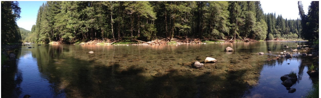
Panorama from right bank showing all 8 structures
