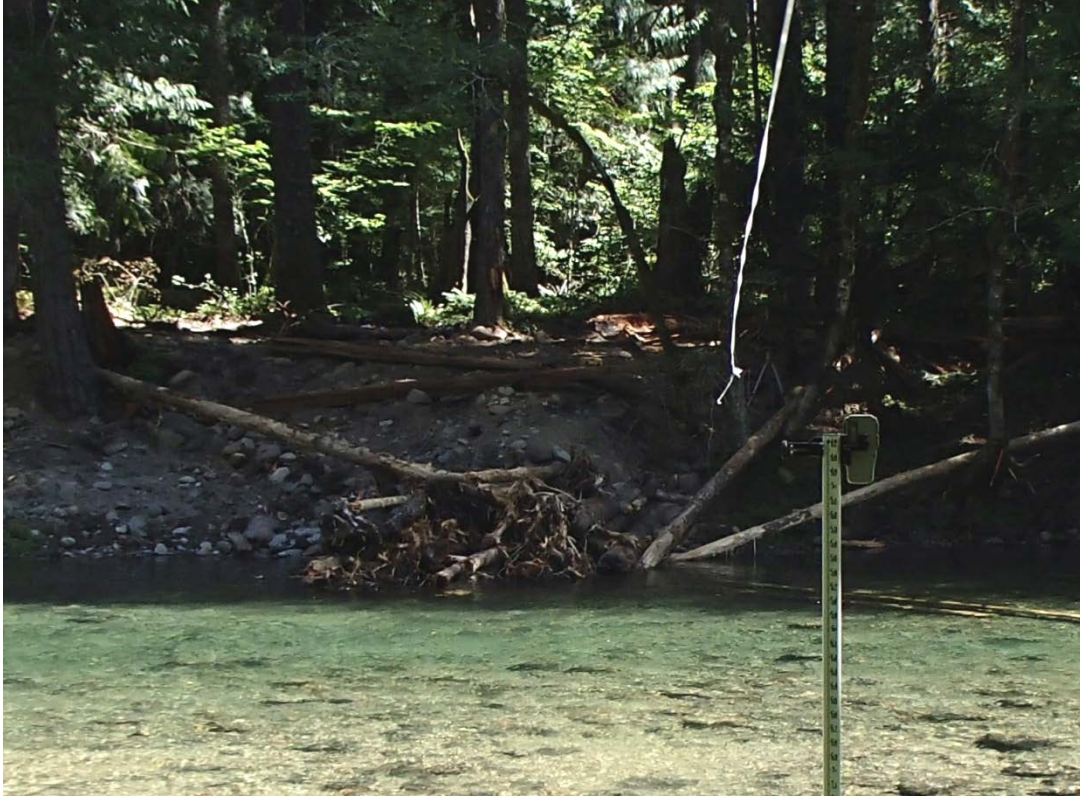
Structure 7 - Looking right bank to left bank
