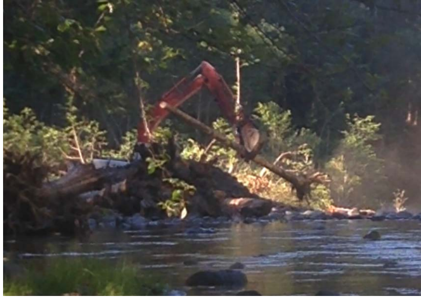
Excavator creating apex log jam
