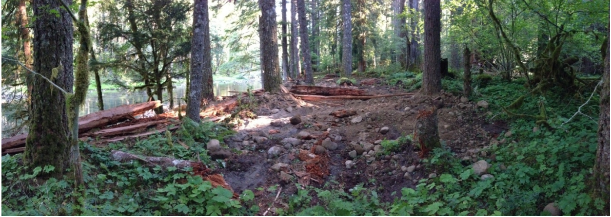
Top of river bank after installation of structures, trenches have been backfilled to maintain level ground
