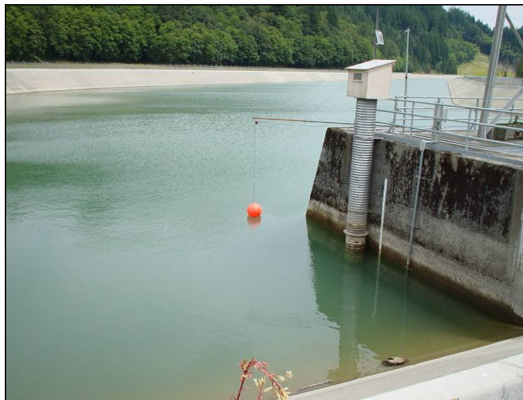
Figure 9. The Swift No. 2 project forebay water temperature monitoring site.
