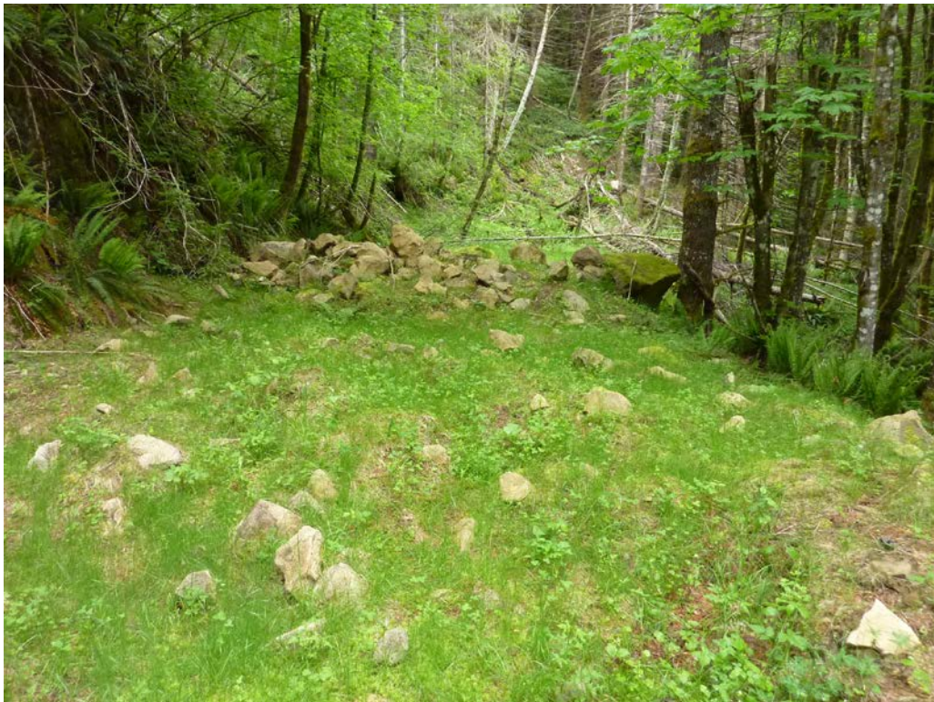
Looking south from the barrier to the slope failure along 7901 Rd.
