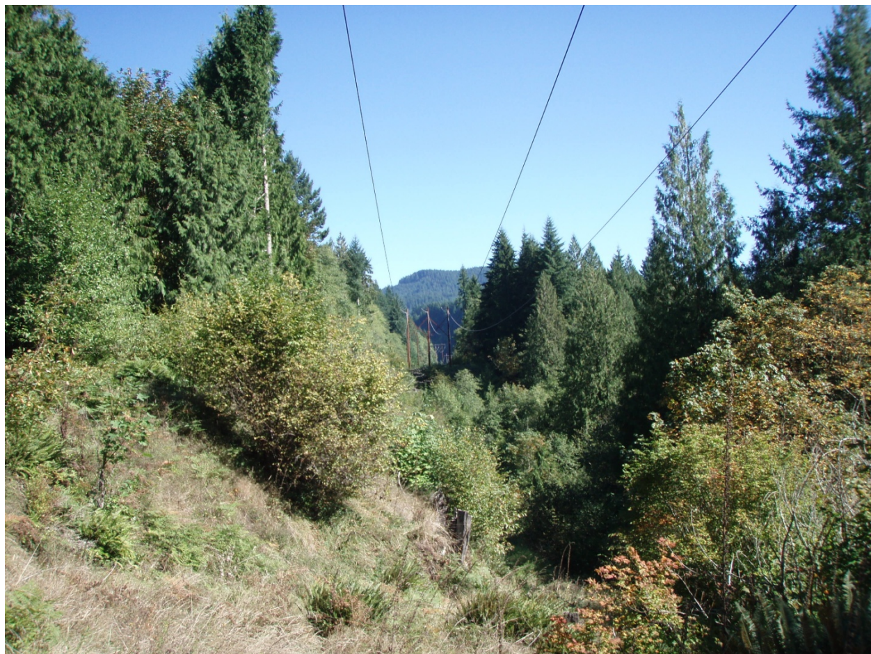
Figure 5: Lake Line 4/10-5/10 shows an example of smaller shrubs becoming a potential hazard because of topography.
