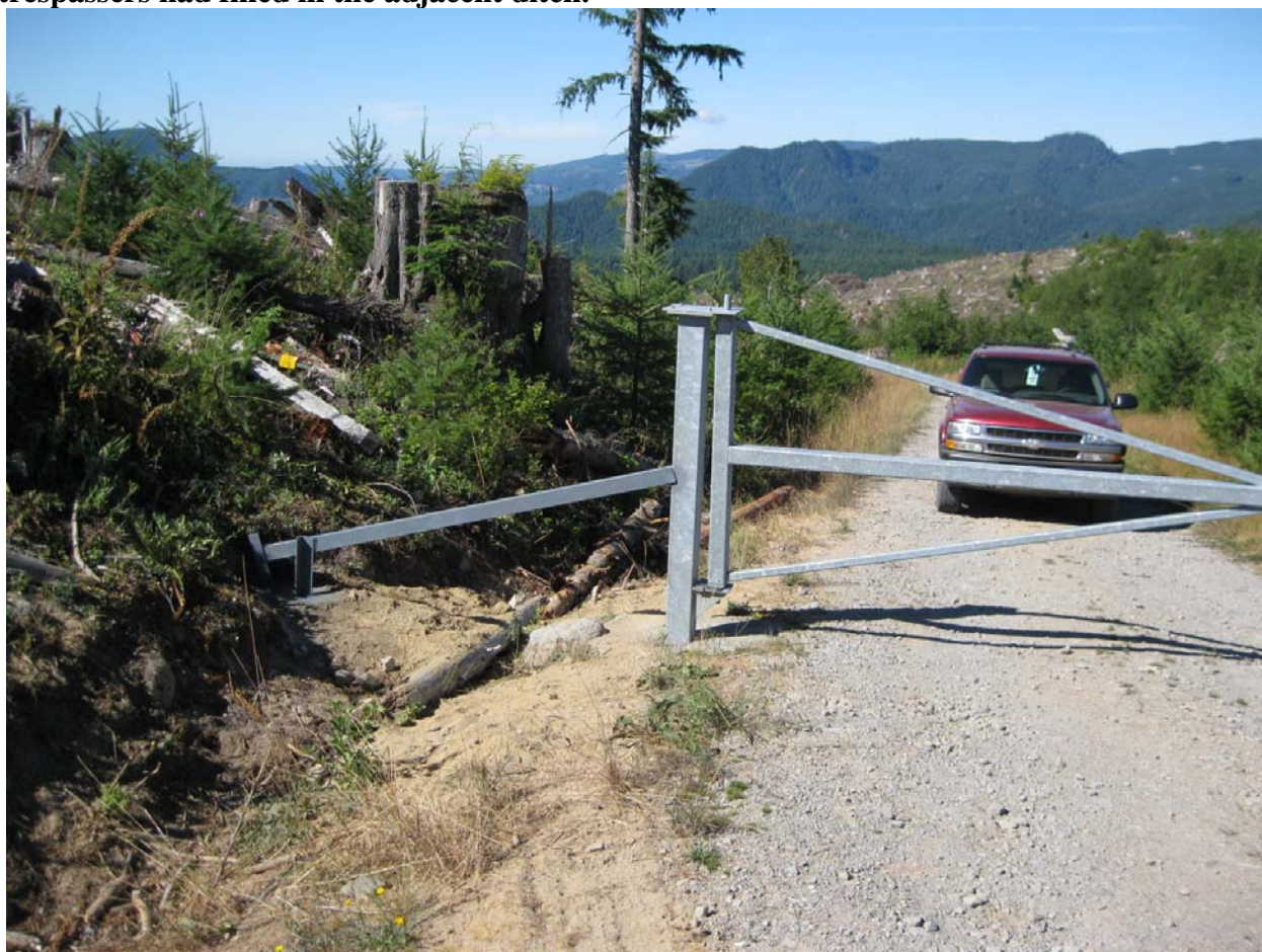
Figure 10. PacifiCorp added extensions to the gate in Management Unit 33 where trespassers had filled in the adjacent ditch.
