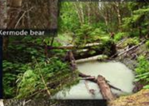
Completed spawning channel
