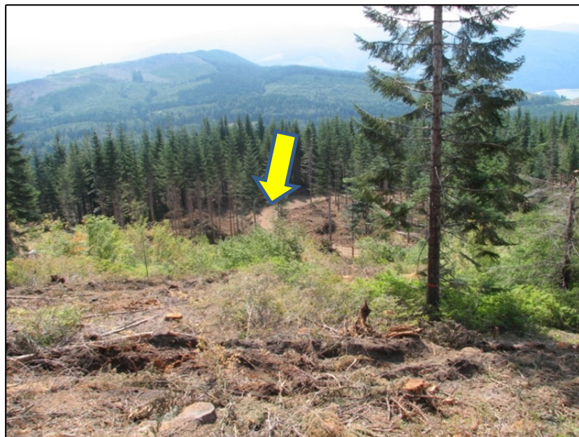
New road (yellow arrow center) built through harvest area in Unit 35.
