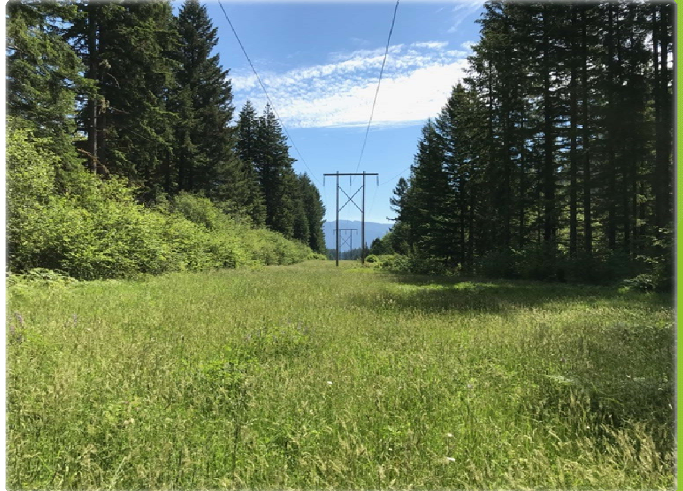
Transmission Line, Looking East
