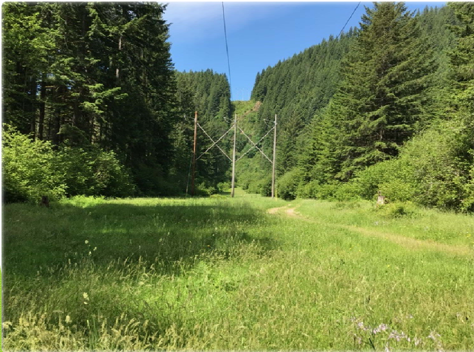
Transmission Line, Looking West
