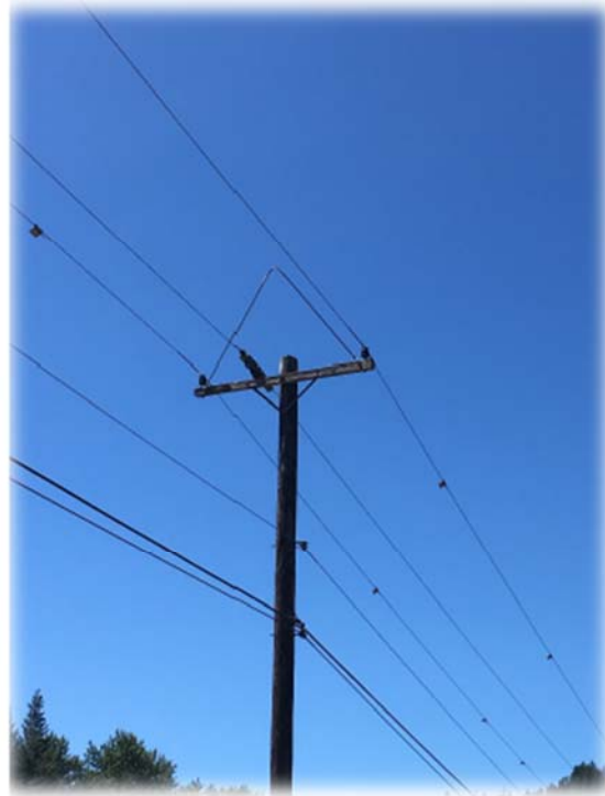
Completed installation of a perch discourager.
