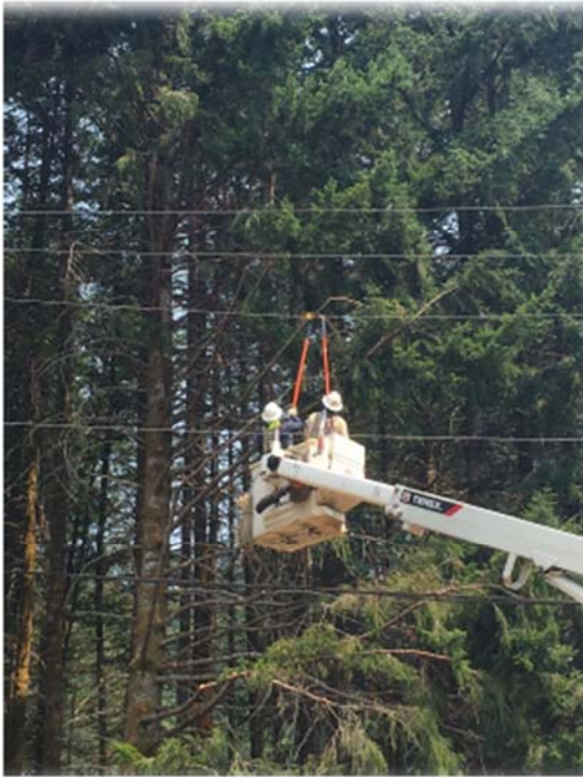
PUD crews installing avian flight diverters.
