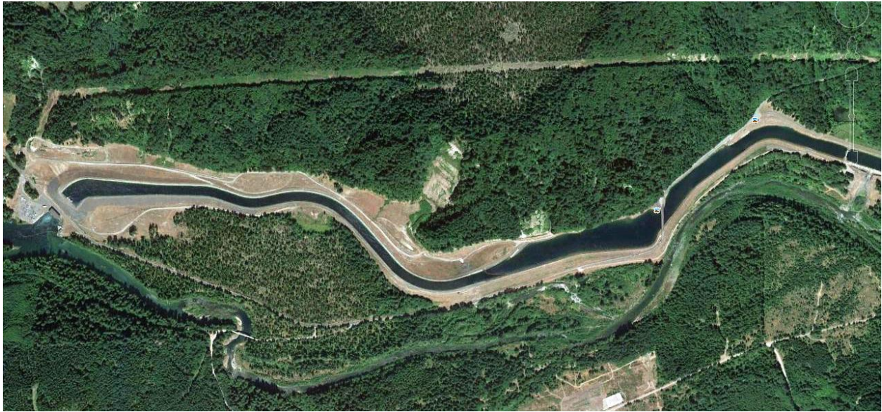
Figure 3.2-1 Project Works Management Unit (Google Earth, August, 2012).
