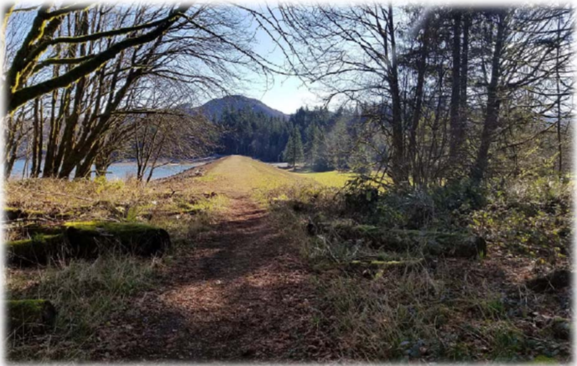
Saddle Dam – North Abutment
