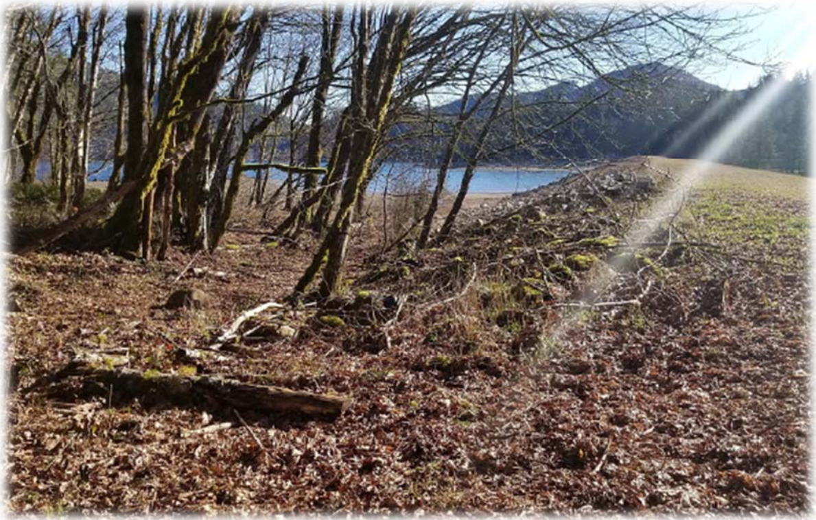
Saddle Dam – East side of North Abutment
