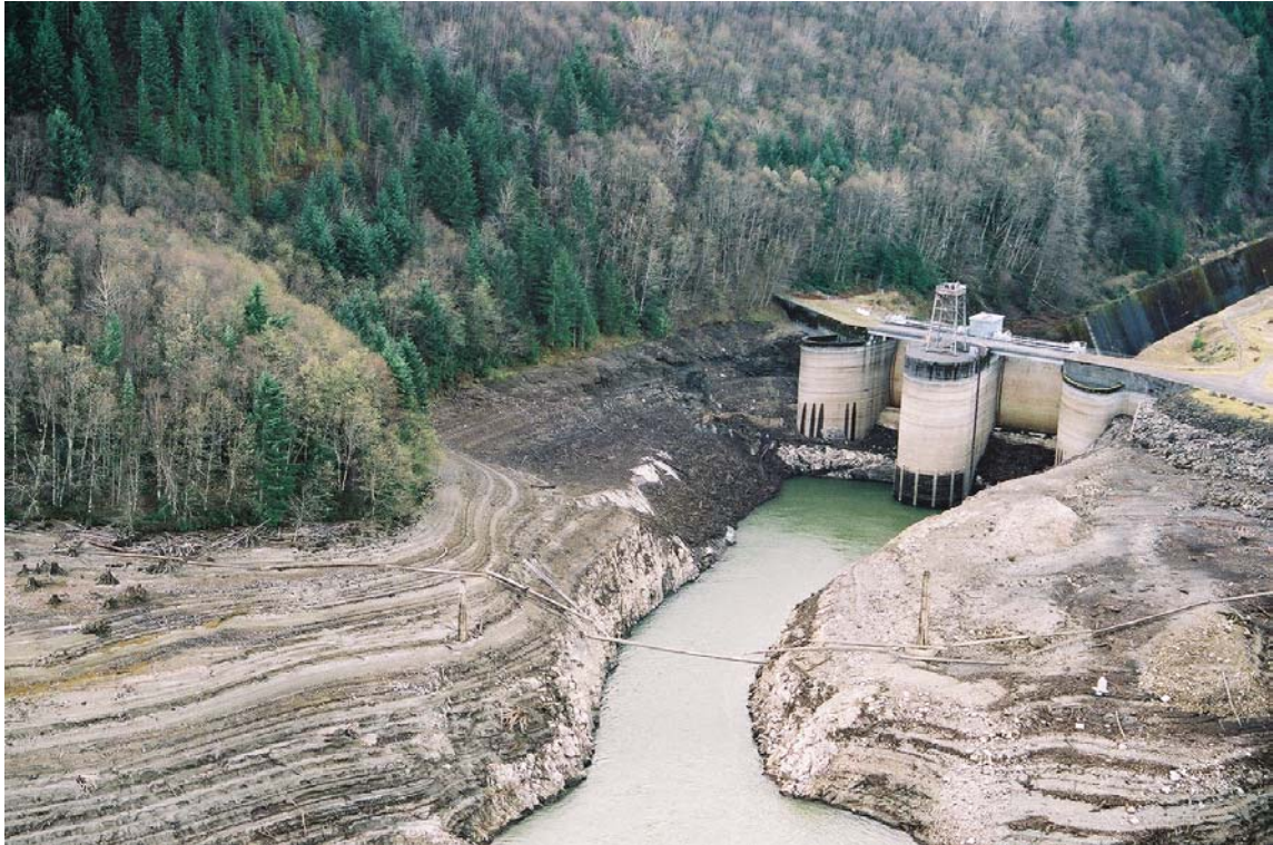
Figure 4.17-2. View of Swift No. 1 Dam displays the two taintor gates and central intake tower.
