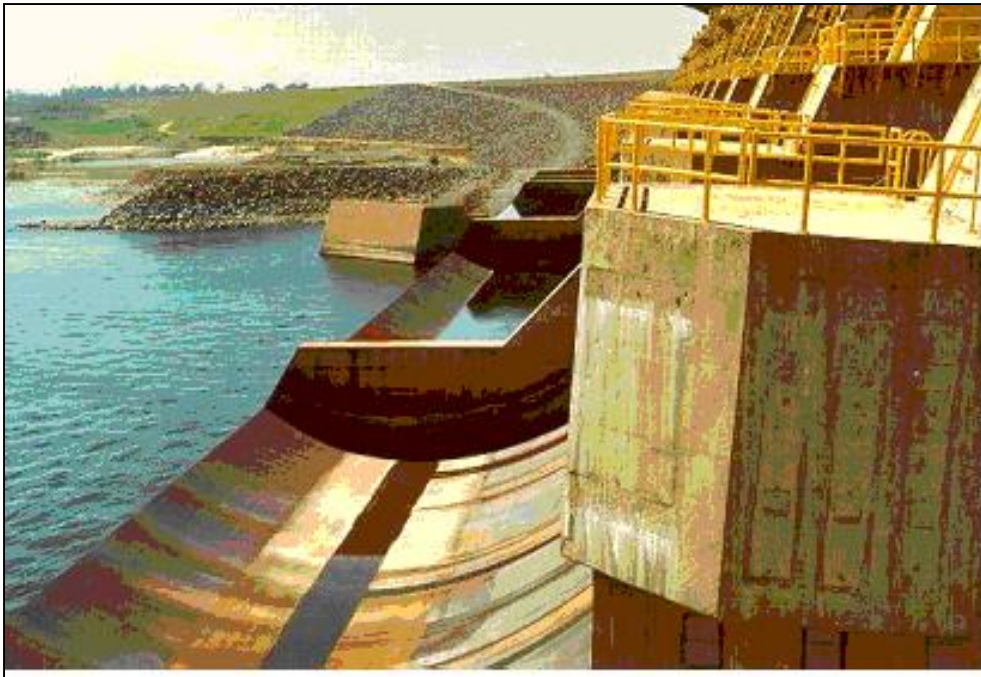
Figure 7. Full flip lip bucket-type spillway.
