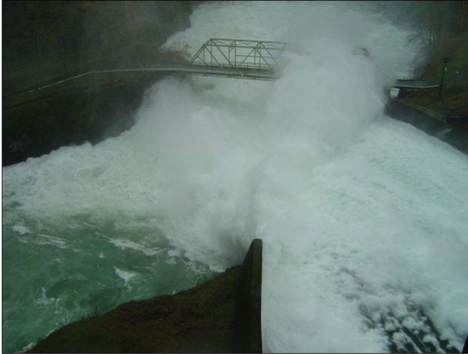
Figure 5: Merwin spill as it exits and oversprays the access bridge.
