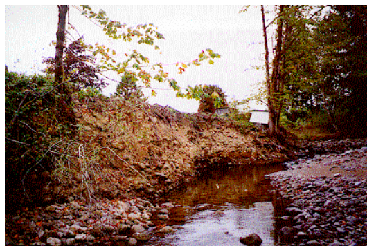
Erosion upstream of Speelyai canal diversion
