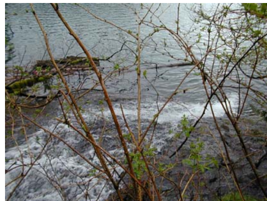
Photo looking downstream of culvert m170c4
