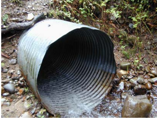
Photo of culvert m170c4 inlet
