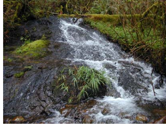
Photo looking upstream of culvert m170c4
