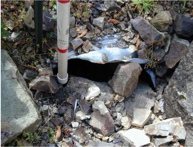
Figure 5.7-6. Culvert with a rusted, crushed, and plugged outlet.
