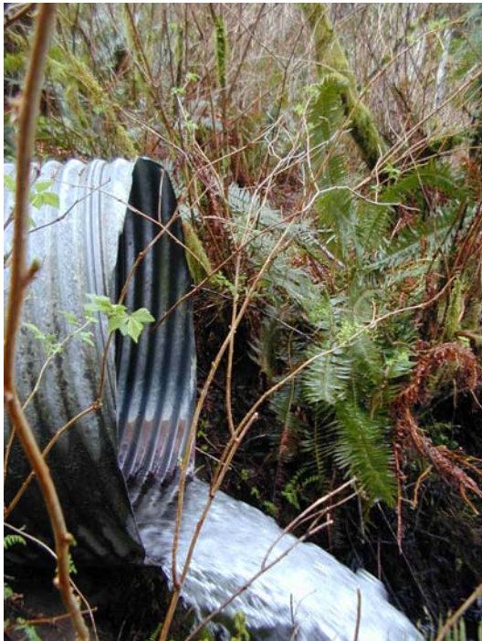
Photo of culvert m170c4 outlet
