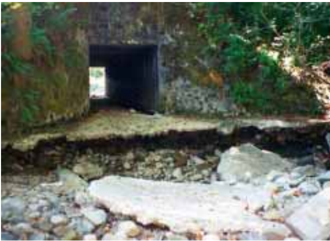
Photo 7. Culvert located within the dry channel segment of Dog Creek, Sept. 10, 1996.
