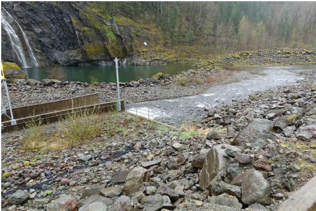
Figure 6. Swift bypass reach (looking downstream from the flow control structure).
