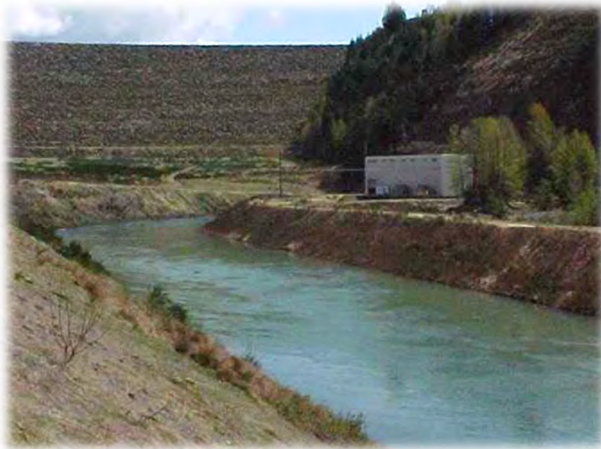
Figure A.3.1-1. Swift Dam, Swift No. 1 Powerhouse, and Swift No. 2 Canal
