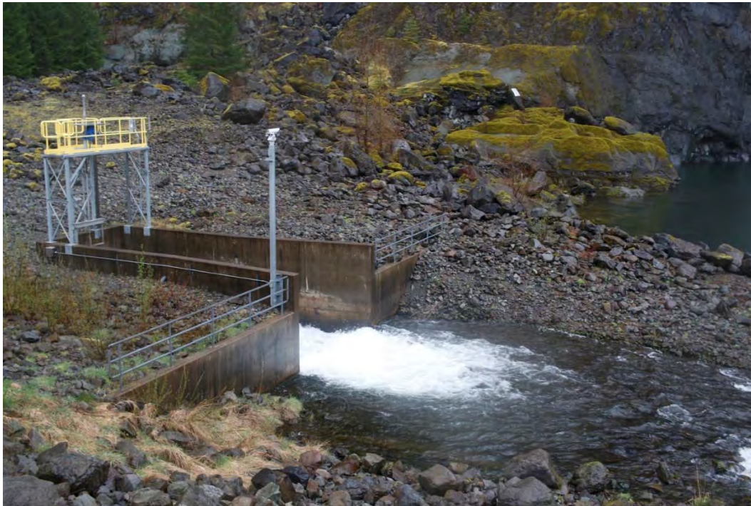
Figure 7. Swift bypass reach (looking upstream from the flow control structure).
