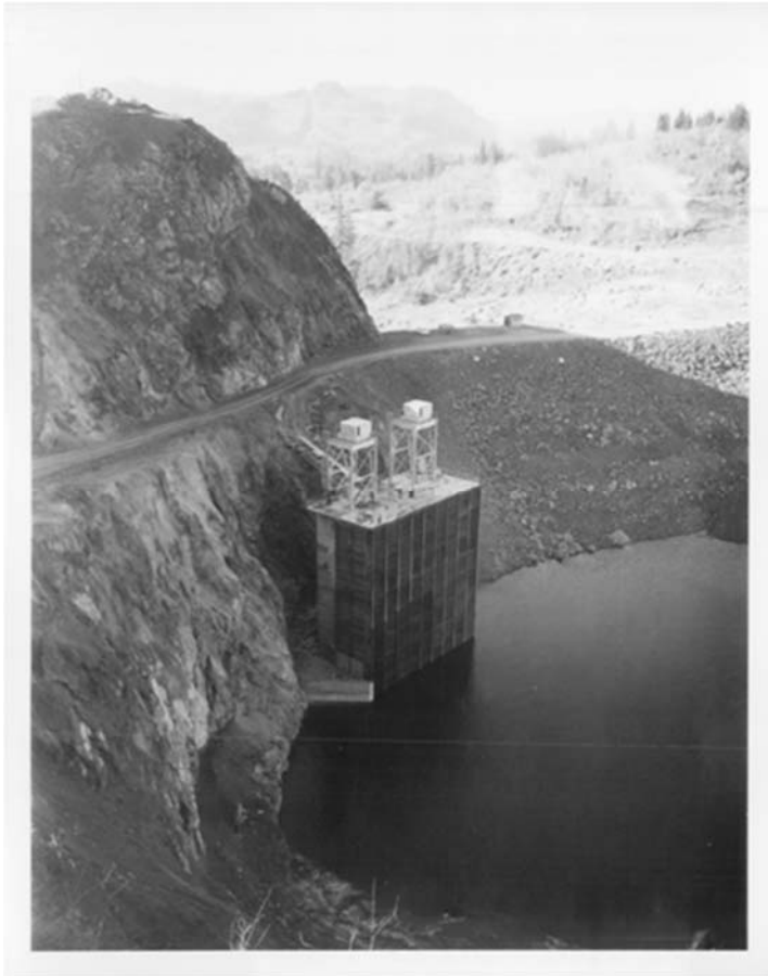
Figure 12. Yale hydro intake structure at low pool during construction.
