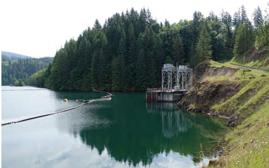
Figure 11. Yale hydro intake structure at high pool.
