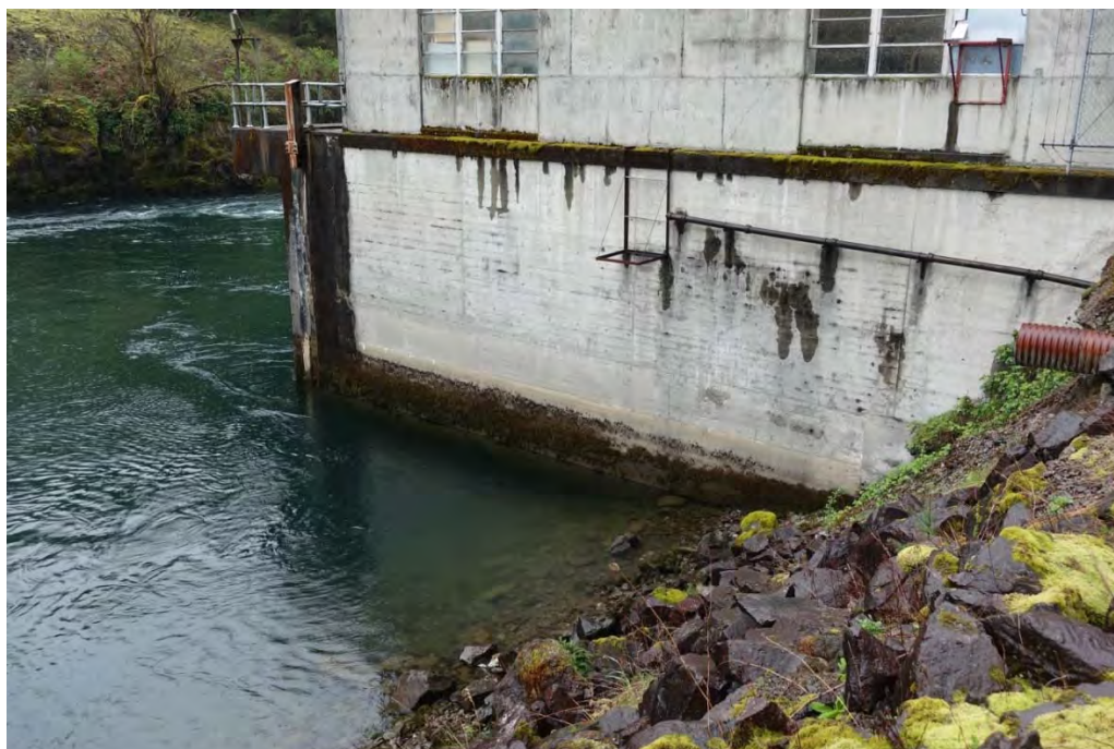
Figure 4. Downstream wall of Yale Powerhouse.
